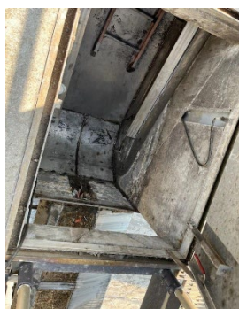
Left: Scum beach being repaired, Right: 3" trash pump used for proof-of-concept testing
