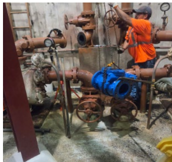
Lakeshore Global Corporation Millwrights replaces the dewatering pump at Bluehill
