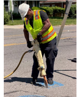
Craig Steele uses jack hammer to break up cement to locate valve
