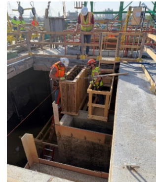
Contractor installing tie rods and formwork for hanging infill wall in Aeration Deck No. 3
