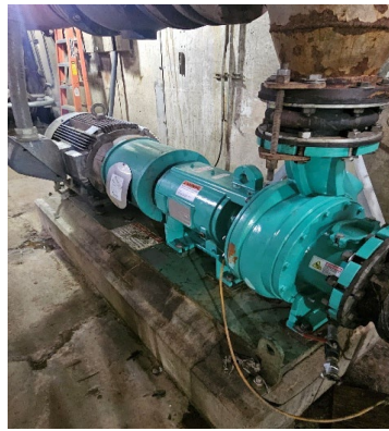
Middle: New pump installed
