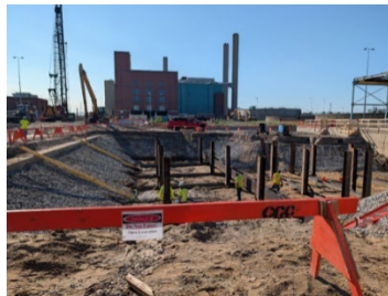
Excavation for the New Grit Processing Facility
