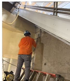
Structure repairs at South Dry Well
