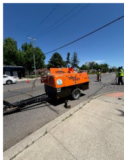
Air compressor is used to power the jack hammer used to break up the cement
