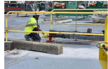
Damaged existing plank removal at AB No. 3
