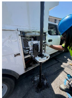
Charles Drayon uses valve turner on box truck to automatically turn valve
