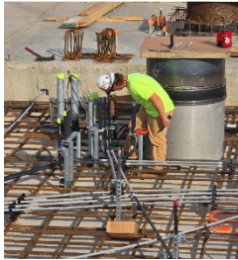
Laying electrical conduit for the new SFE Building
