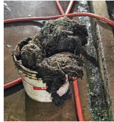
Right: Raas removed from the SFP #1
