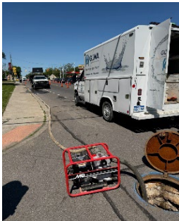
Water pump used to drain water from the manhole in order for crew member to go inside the manhole to correctly measure the location of the valve
