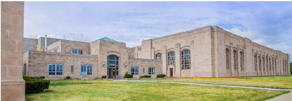
GLWA Springwells Water Treatment Facility
