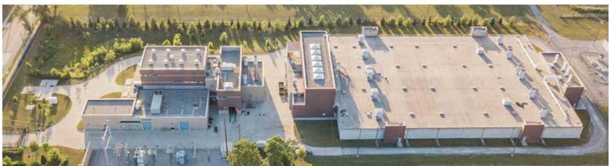
GLWA Hubbell-Southfield Facility
