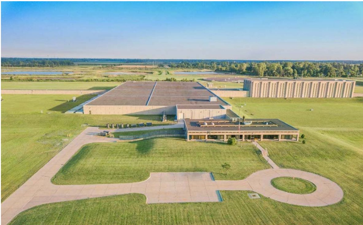
GLWA Lake Huron Water Treatment Facility
