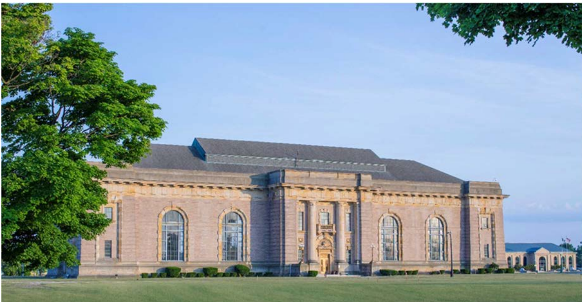
GLWA Water Works Park Water Treatment Facility
