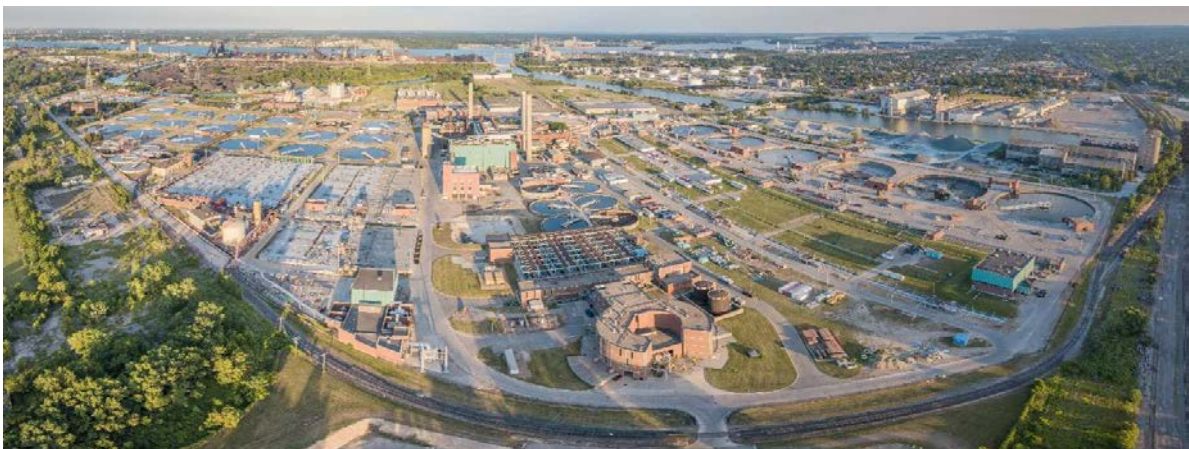
GLWA Water Resource Recovery Facility
