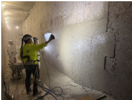
Waterproofing the flow channel walls
