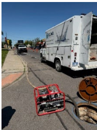
Water pump used to drain manhole
