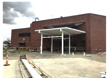
Ragland Canopy Installed
