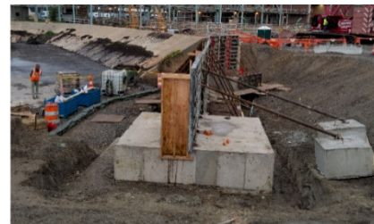
Ash Lagoon Concrete Work Progress
