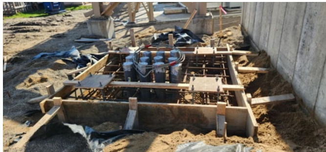
Foundation structural support for conduct
