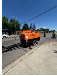
Air compressor for powering jack
