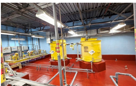
After: Containment area
