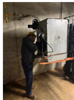
Jamen Burgess, Maintenance Technician
