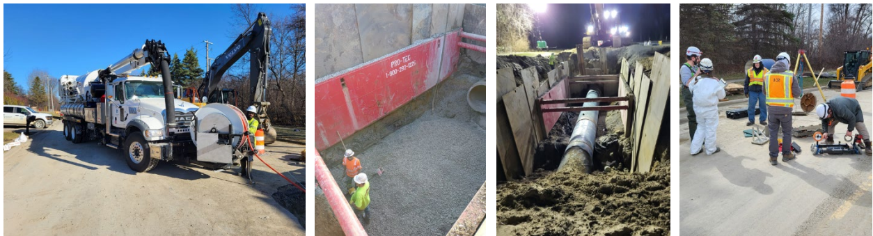
GLWA Maintenance and Repair team assisting with cleaning the 48-inch water main, additional pipe segment installation and replacement, and the HDR pipeline inspection team
