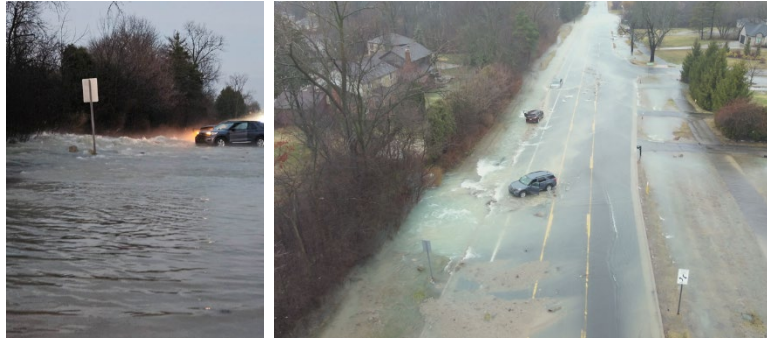
14 Mile Road 48-inch water main break
