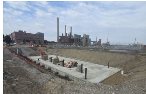
New concrete foundation over West effluent channel
