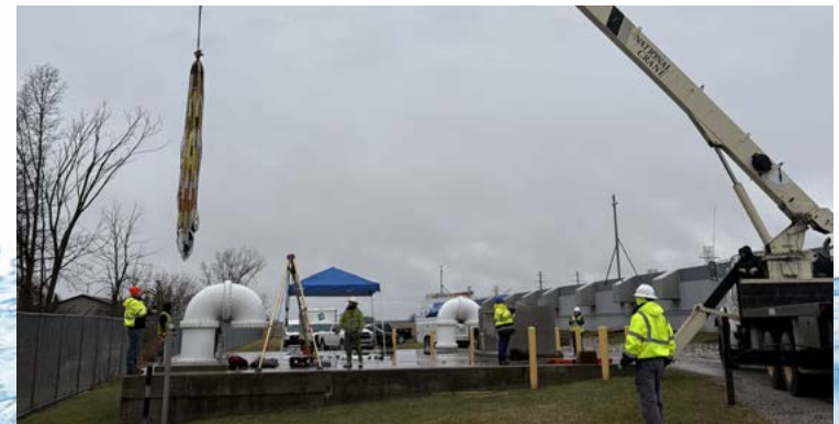
Inspection Tool Removal at Imlay City Booster Pump Station
