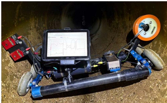
Electromagnetic Inspection in the 14-Mile Road Transmission Main
