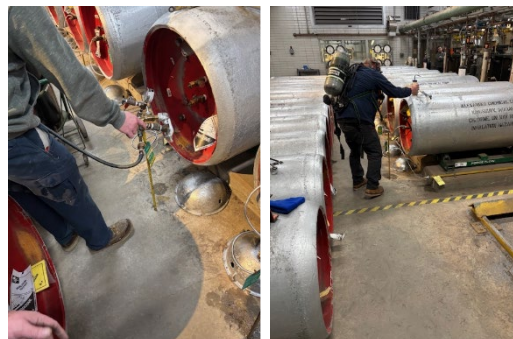
Terry Helmold, Jamen Burgess, and Jacob Falter performing flex line changes
