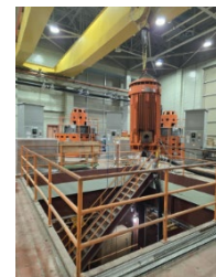
Sanitary Pump 10 at Freud SPS being lifted
