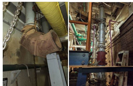
Sections of ash system piping were replaced in the basement and on the 4th floor of Complex II Incineration.
