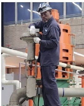
Robert Oliver Jr. disassembling a vacuum breaker
