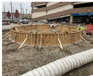
Seat Wall Concrete Installed
