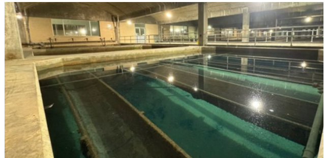
CIP project highlighted at the Charges Rollout 1 and 2 meeting of a view of the existing filter beds at the Northeast Water Treatment Plant that will be replaced as party of CIP Project #112008
