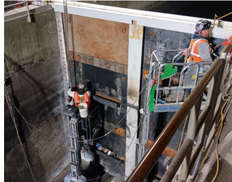
Effluent Channel Bulkhead Installation
