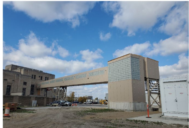
CIP project highlighted at the Charges Rollout 1 and 2 meeting of a utility bridge constructed at the Springwells Water Treatment Plant providing access to electrical systems that feed pumping operations
