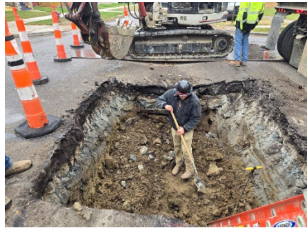
Excavating and investigating sunken pavement at Third Street and Webb Street in the City of Detroit
