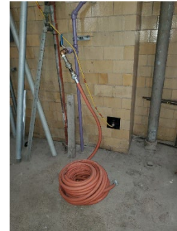
Temporary air hose connected to pneumatic system
