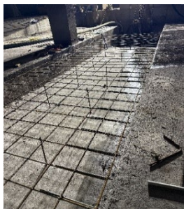
Center sump channel filled in with concrete to form flat area for future cleaning
