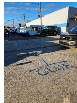
Inspector Troy Davenport marking GLWA's 54-inch water main at 16153 Garfield Street, Detroit
