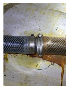
The new barbed PVC coupling and titanium worm-gear hose clamps
