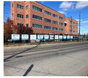
Jefferson Signage Relocated to Fence
