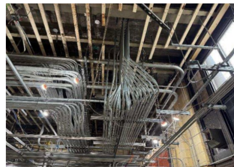
Conduits installation in the Monitoring Room
