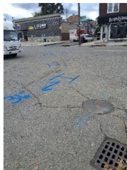
Inspector Dwayne Pittman marking GLWA's 36-inch water main at 2217 Springwell Street, Detroit
