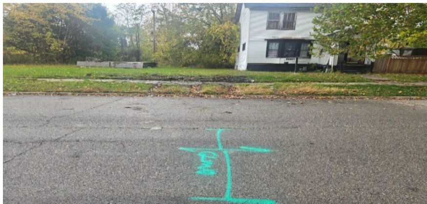
Inspector Tammie Dubose marking GLWA's 16-inch sewer main at Manistique Street, Detroit
