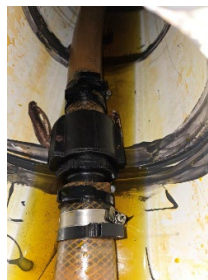
The old camlock coupling with the nylon hose clamps
