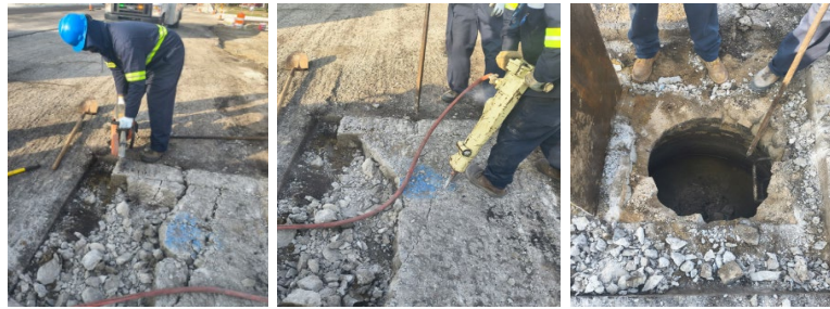
Saw cutting and jack hammering pavement to successfully locate buried access hatch and air release valve on 14 Mile Road
