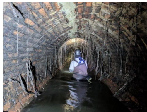
CIP Project #250210 – Rehabilitation of GLWA Sewers, Ashland Relief, Linwood, Lonyo, Second Avenue, and Shiawassee – Winning photo by Greg Marker
