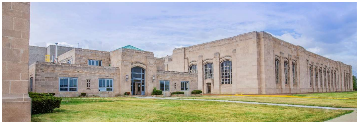
GLWA Springwells Water Treatment Facility
