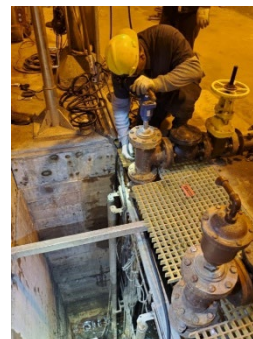
Maintenance team member installing new sump pumps
