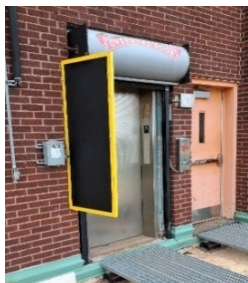
Sunscreen installed to mitigate the sun's impact on the elevator sensors
