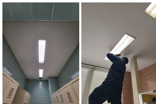
Southwest second floor ceiling painted, and light fixtures cleaned, Electrician Thomas Medici pictured
