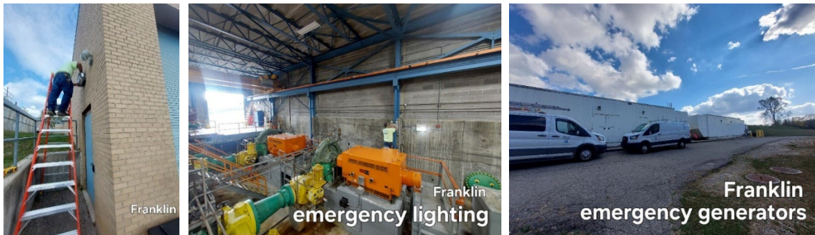
Exterior fixtures and emergency lighting batteries being replaced at Franklin Station (Thomas Medici in photos)
