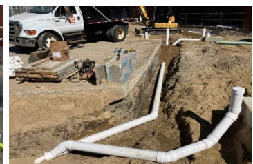
Ragland canopy footing installation
