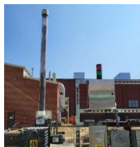
New indicating light installed at grit channel no. 4N
