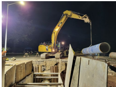
Installing new 42-inch steel water main
