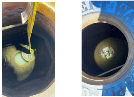
Chlorine introduction point and final access hatch installation of 7 Mile Road and Nevada Street water main
