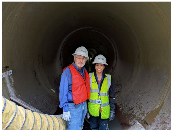
Tom Hall and Mini Panicker in the Newly Installed HOBAS Pipe at Fox Creek
