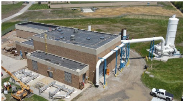
Aerial view of OMIDDD's newly constructed electrical building at the Northeast Sewage Pumping Station (NESPS)
