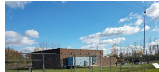
Figure 38. Ypsilanti Pump Station
