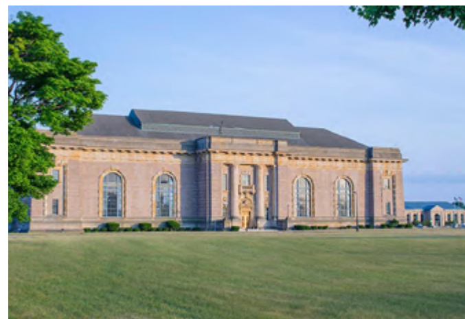
Figure 10. Water Works Park WTP
