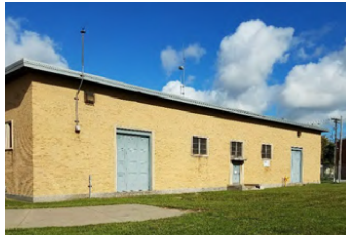
Figure 21. Eastside Pump Station
