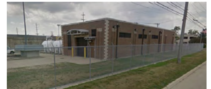
Figure 35. Schoolcraft Pump Station
