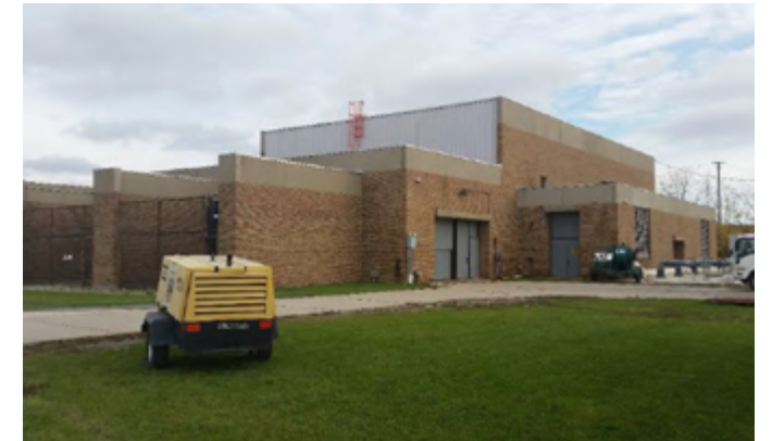
Figure 61. Northeast Pump Station
