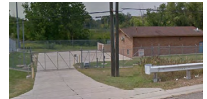
Figure 32. Orion Pump Station
