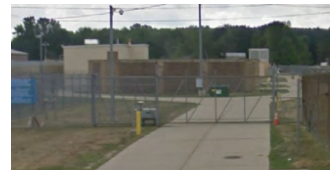
Figure 27. Joy Road Pump Station
