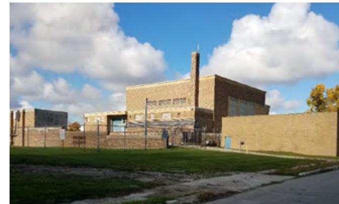
Figure 59. Freud Pump Station
