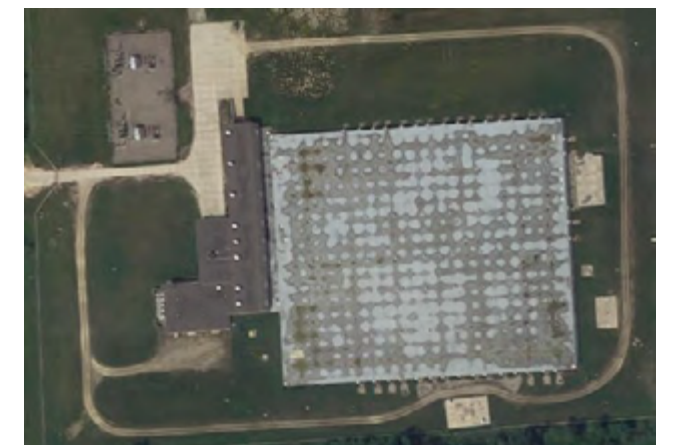
Figure 28. Imlay Pump Station
