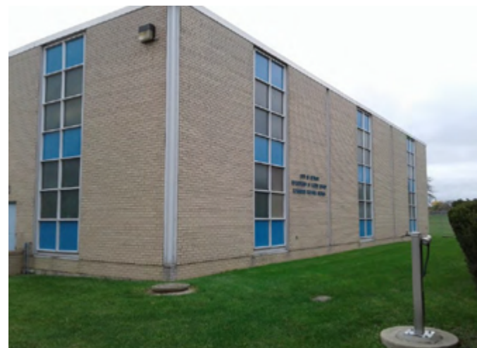
Figure 29. Newburgh Pump Station
