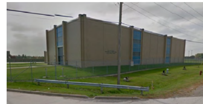
Figure 31. North Service Center
