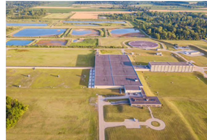
Figure 3. Lake Huron WTP
