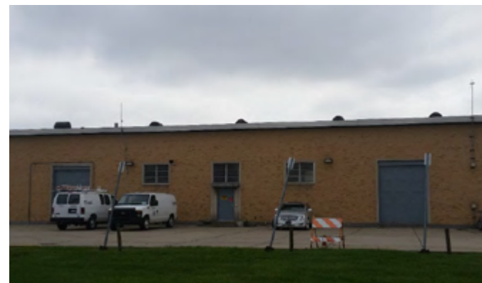
Figure 30: Northwest Pump Station
