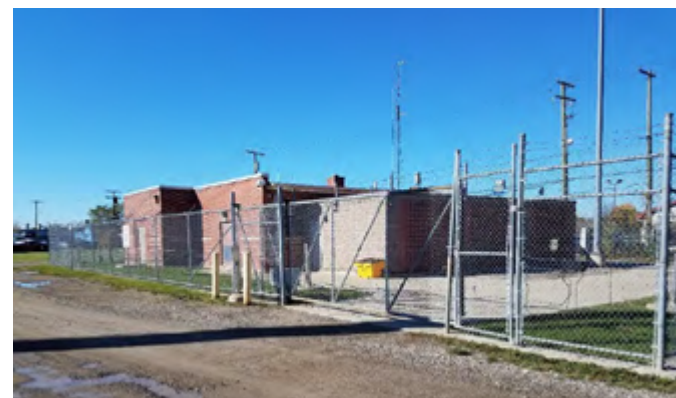
Figure 26: Michigan Avenue Pump Station
