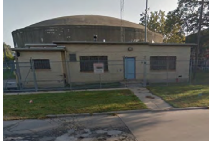
Figure 22. Electric Avenue Pump Station
