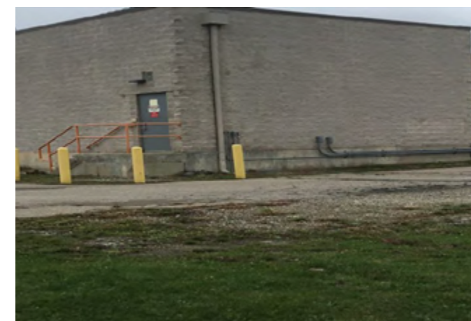
Figure 20. Adams Road Pump Station
