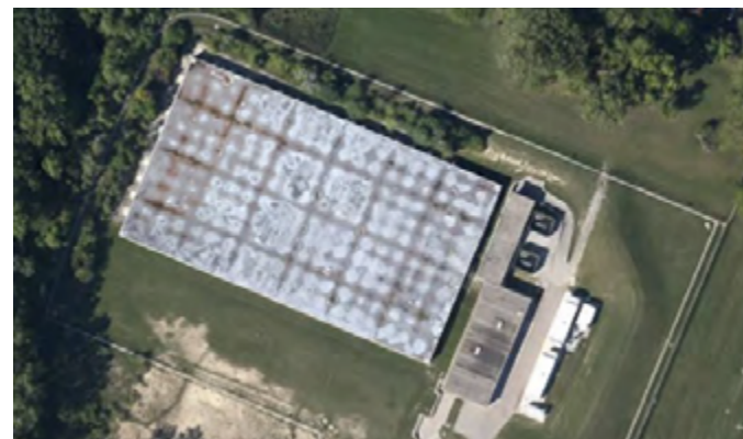
Figure 25. Franklin Pump Station
