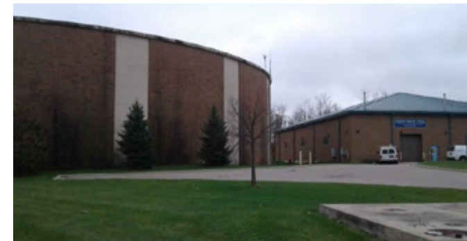
Figure 23: Haggerty Pump Station
