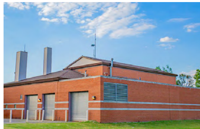
Figure 43. Puritan-Fenkell CSO RTB
