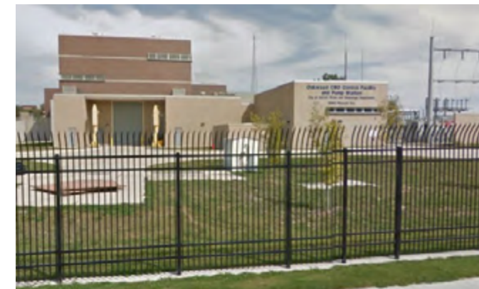
Figure 62. Oakwood Pump Station
