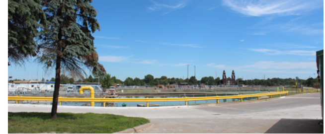
Assessment and Rehabilitation of WRRF yard piping and underground utilities
