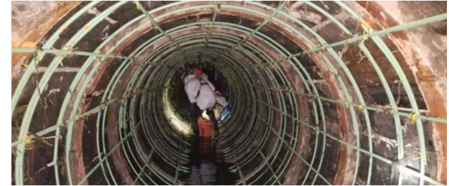
CON-149, Emergency Sewer Repair
