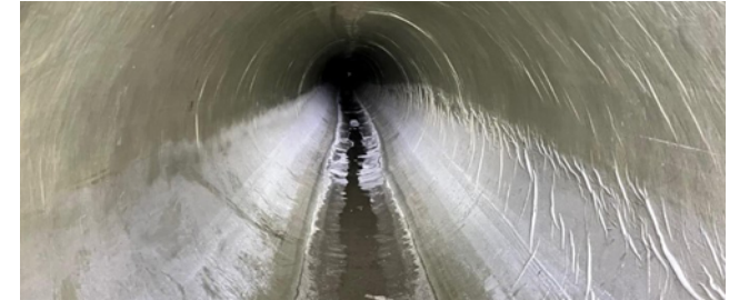
Sewer Rehabilitation and Repair
