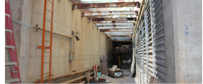
WRRF Structural Improvements
