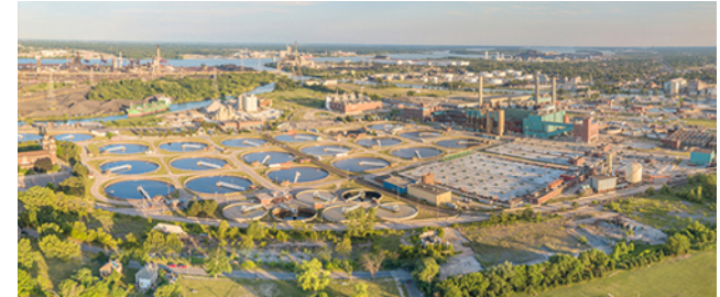
WRRF Rehabilitation of the Secondary Clarifiers Phase 1
