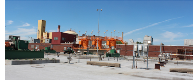
WRRF Aeration Improvements 3 and 4
