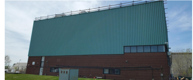
2022 WRRF Roof Improvements Project
