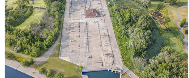
Hubbell Southfield CSO Facility
