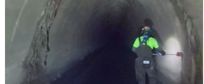
Conveyance System Repairs (Sewers)
