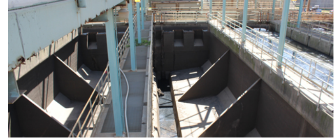
WRRF PS #2 Bar Racks Replacements and Grit Collection System Improvements
