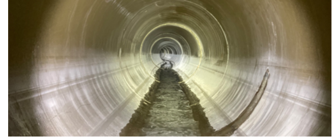
B-39 Outfall Rehabilitation
