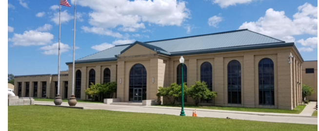
Masonry Replacement and Rehabilitation Program
