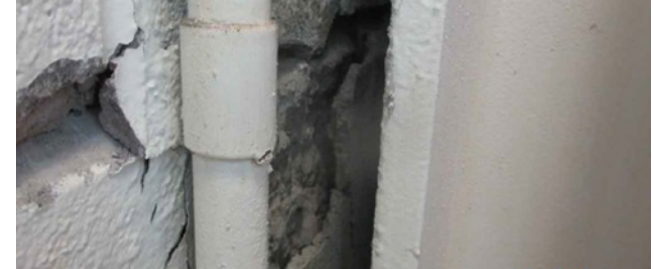
Structural Inspection and Structural Improvements
