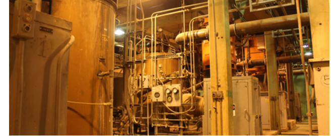
Rehabilitation of Screened Final Effluent (SFE) Pump Station
