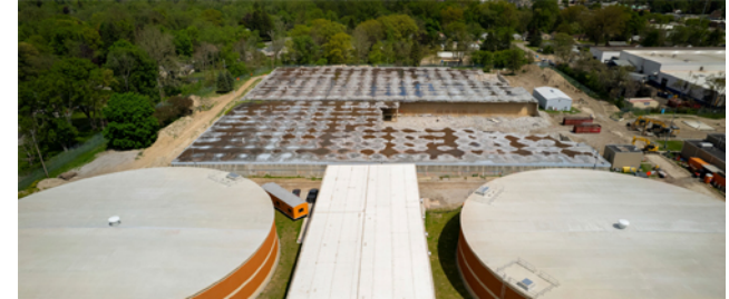
West Service Center Pumping Station
