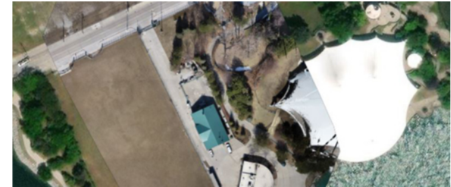
CSO Facilities Improvements II
