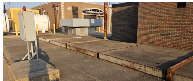
Schoolcraft Pumping Station
