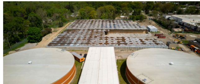
West Service Center Pumping Station
