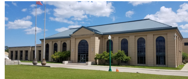
Water Works Park Water Treatment Plant
