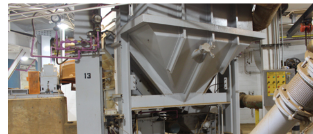
WRRF Rehabilitation of the Ash Handling Systems
