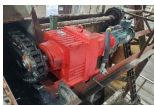
New gearbox installed
