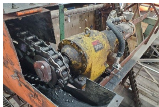
Old gearbox before replacement
