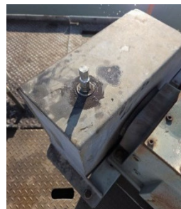
Oiling port installed on the top of a drive chain shroud for Secondary Clarifier No. B-2
