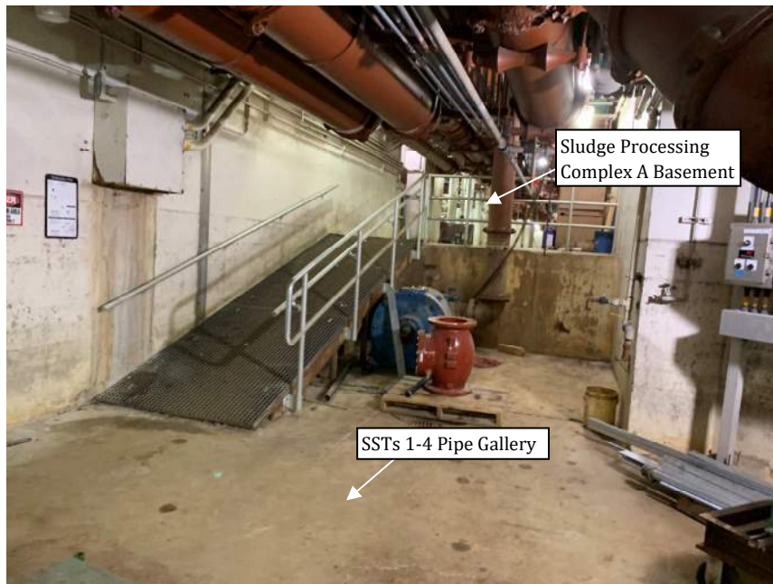
Figure 3-2: Ramp from SSTs 1-4 Pipe Gallery to Sludge Processing Complex A Basement
