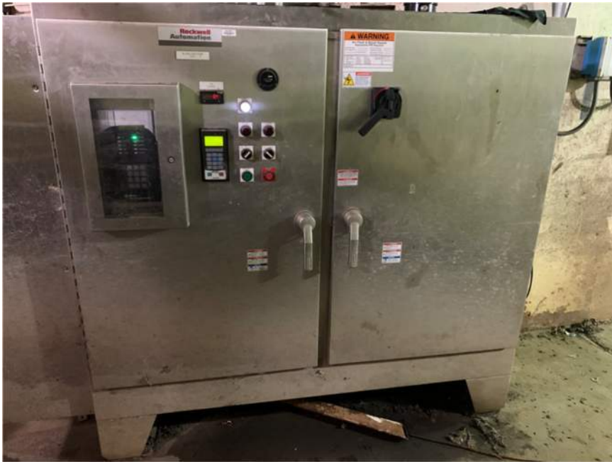
Figure 6-11: SFP-1 VFD
