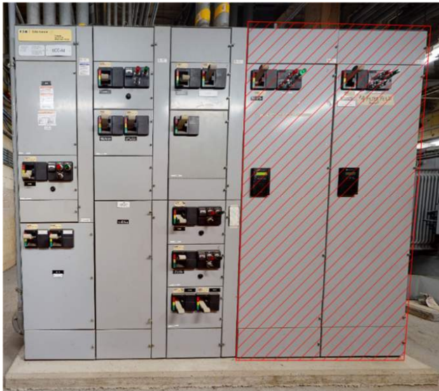
Figure 4-7: MCC-A4 Vertical Section Demolition
