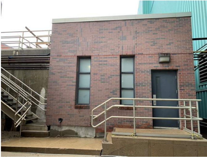
Figure 7-1: SSTs 5/6 Pump Building
