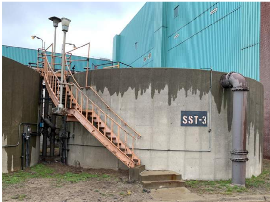
Figure 4-1: Sludge Storage Tank 3 (typical of SST 1-4)
