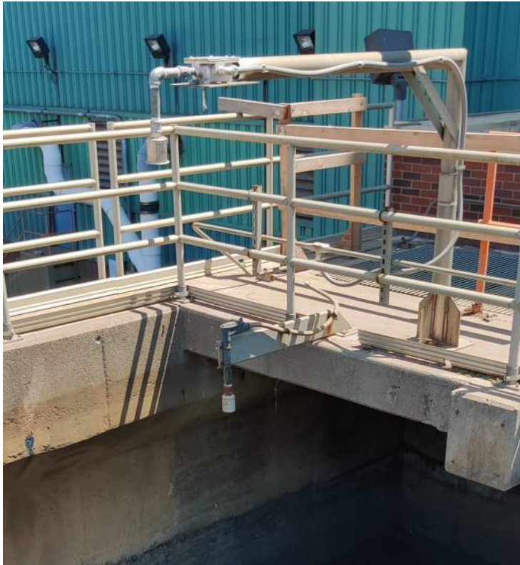
Figure 5-6: SST-6 Level Sensors
