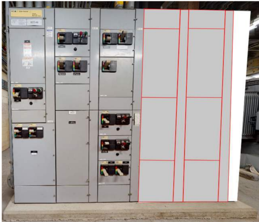
Figure 4-8: MCC-A4 Vertical Section Additions
