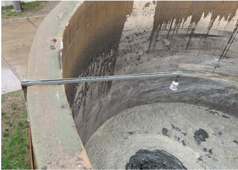
Figure 4-6: Typical SST 1-4 Ultrasonic Level Sensor
