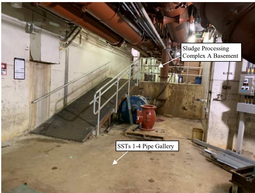
Figure 6-2: Ramp from SSTs 1-4 Pipe Gallery to Sludge Processing Complex A Basement
