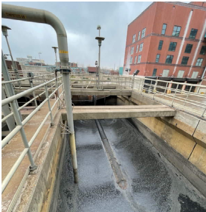
Figure 5-1: Sludge Storage Tank 6
