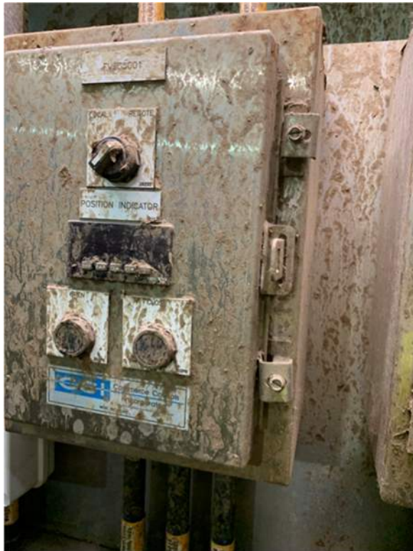
Figure 7-11: Sludge Covering Control Station
