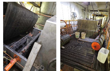
J-conveyor head pulley is removed, and the new head pulley staged for installation as shown in the left and right photos above
