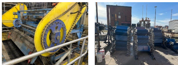
The new drive shaft, sprockets and chain on Bar Rack #3 and the buckets and chain are being prepared for Grit Collector #3
