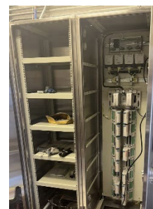
New Network Cabinet (left, devices not installed) and New Controls Cabinet
