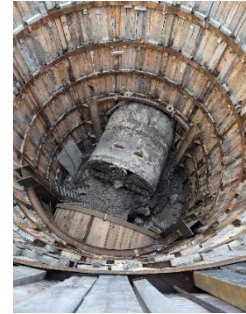
New Tunnel Connecting Fox Creek Enclosure and Manistique Sewer
