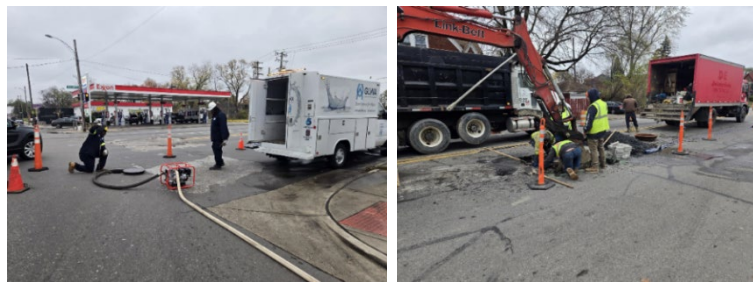
Repairing valves on Schoolcraft Road (left) and repairing and raising buried structures on Schoolcraft Road (right)
