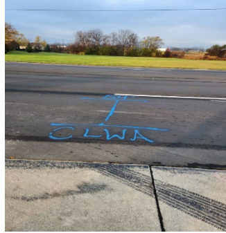
Troy Davenport staked this 54-inch water main at Superior Road and Allen Road (left) and he also staked this 24-inch water main on Eureka Road (right)
