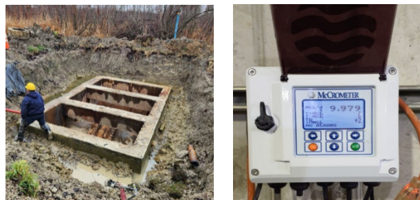
Preparing 96-inch valve vault at Kilgore Road (left) and monitoring flow for 14 Mile Loop (right)
