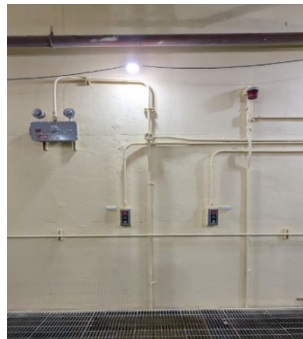
New wall coating at Steady Bearing Floor
