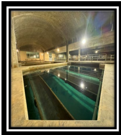
Northeast Water Treatment Plant Filtration Replacement
