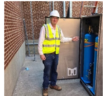
Team Leader Ray Zdonkiewicz is pictured above with the moisture reduction pump provided by SD Myers
