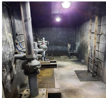
Preventative maintenance at valve remote #15
