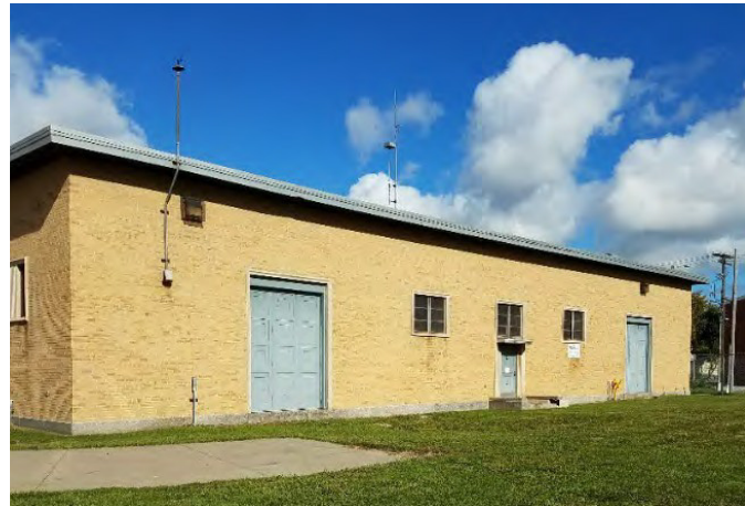
Figure 21. Eastside Pump Station
