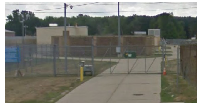
Figure 27. Joy Road Pump Station
