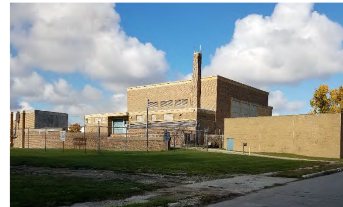
Figure 59. Freud Pump Station
