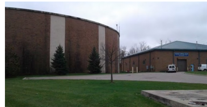
Figure 23: Haggerty Pump Station
