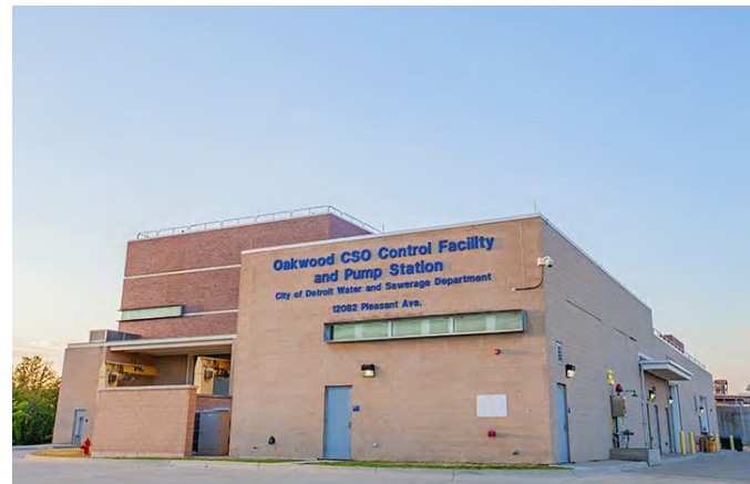
Figure 42. Oakwood CSO RTB
