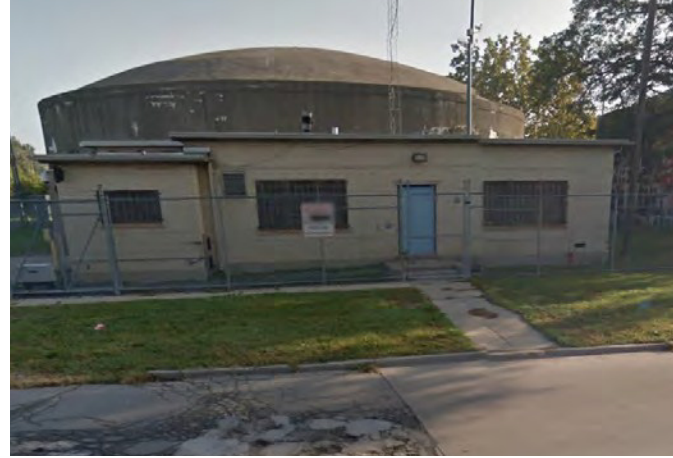
Figure 22. Electric Avenue Pump Station
