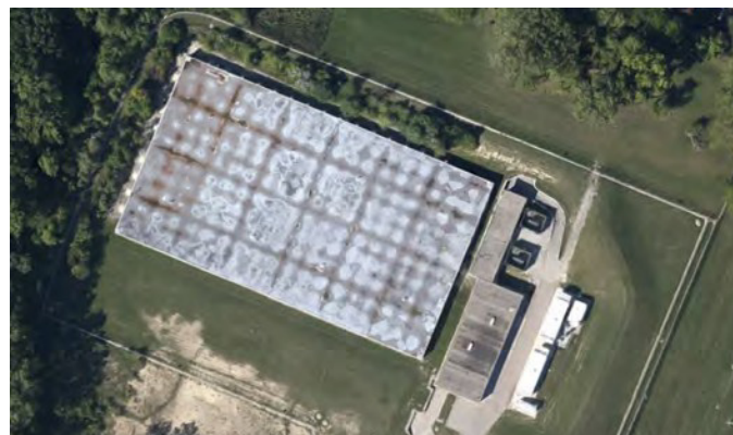
Figure 25. Franklin Pump Station
