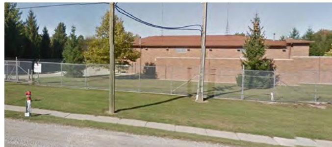
Figure 33. Rochester Pump Station
