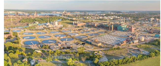
WRRF PS No. 2 Pumping Improvements - Phase 1
