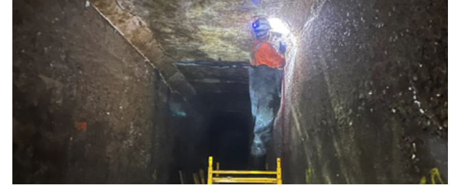
Conveyance System Repairs (Outfalls)
