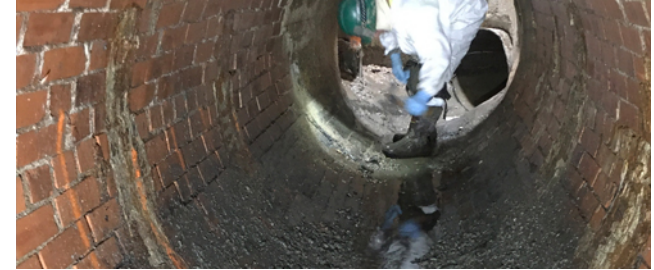
Rehabilitation of Woodward Sewer Systems
