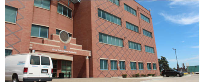
WRRF 4th Floor Renovation
