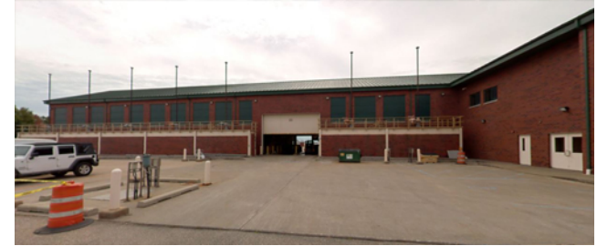
Flushing System Improvements at Conner Creek and St. Aubin CSO Facilities
