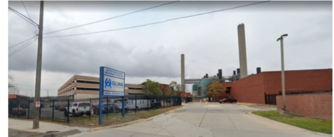
WRRF Front Entrance Rehabilitation
