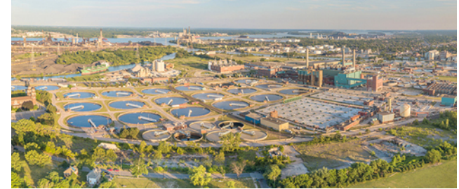
CSO Emergency Generator Improvements
