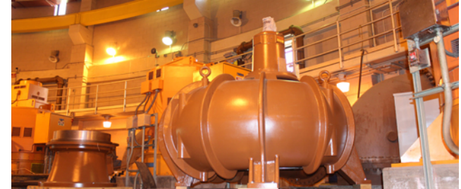
WRRF PS No. 2 Improvements Phase II
