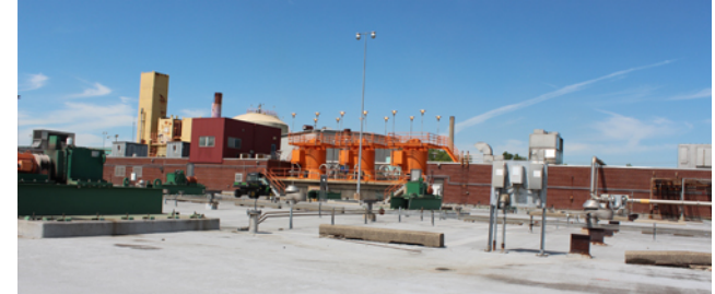
WRRF Aeration Improvements 3 and 4
