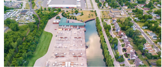
CSO Facilities Improvement Program
