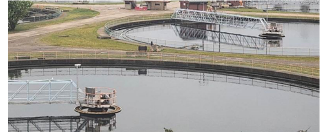
WRRF Rehabilitation of the Secondary Clarifiers
