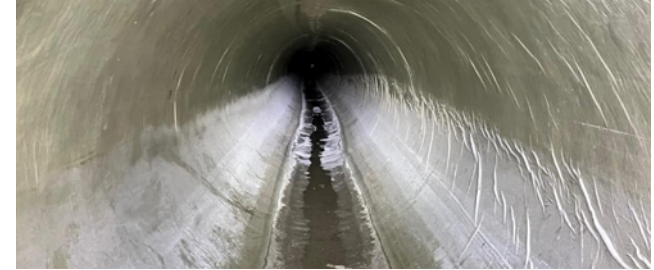
Sewer Rehabilitation and Repair
