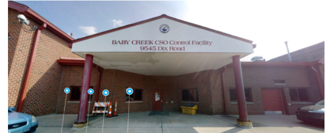
Baby Creek CSO Facility Influent Flushing System
