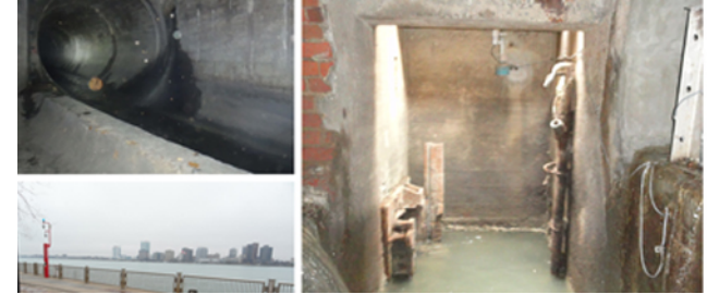
Conveyance System Infrastructure Improvements
