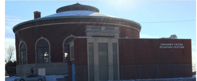
Conner Creek Pump Station Improvements
