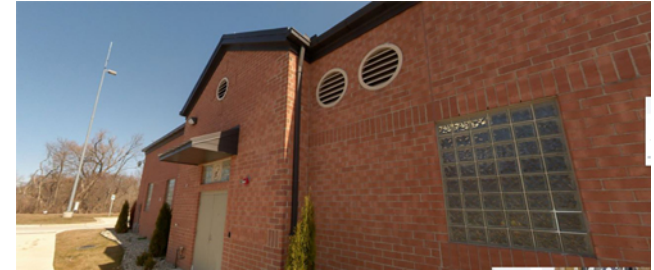
Conversion to Complete Capture Basin at Puritan Fenkell and Seven Mile CSO Facilities
