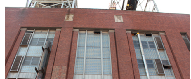
WRRF Roof Replacement for Multiple Facilities Program
