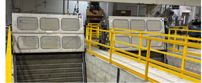
CSO Baby Creek Screen Rehabilitation
