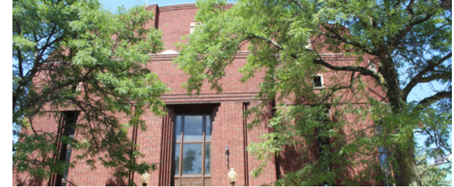
WRRF PS No. 1 Improvements
