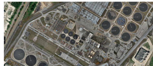
WRRF Roof Improvements - Phase II
