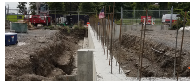
Fairview Pumping Station - Replace Four Sanitary Pumps
