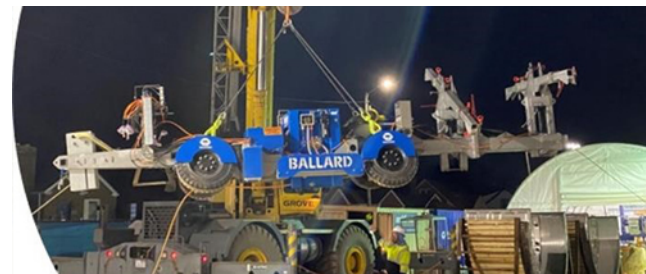
Raw Water Supply Tunnel
