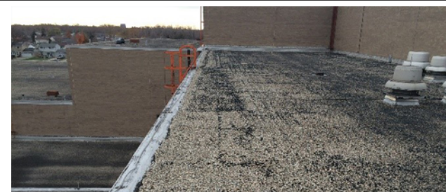
Lake Huron and Southwest Roof
