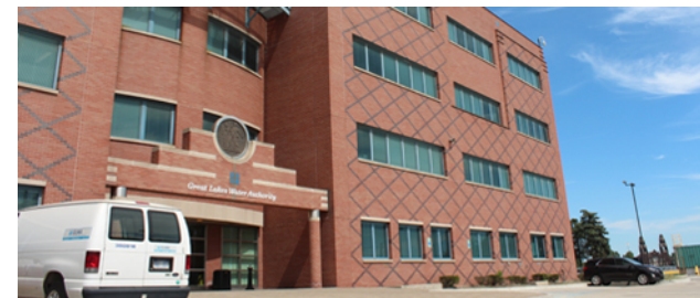
WRRF 4th Floor Renovation
