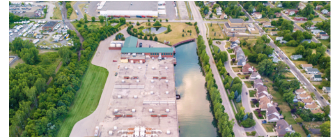
CSO Facilities Improvement Program
