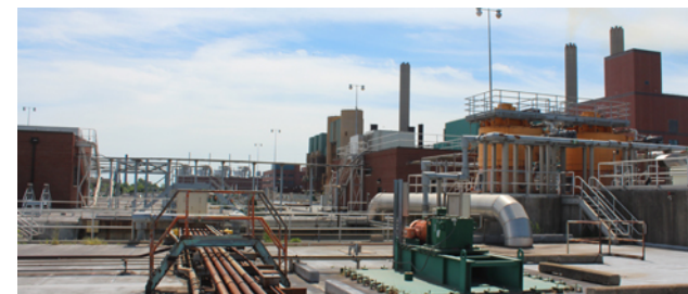
WRRF Aeration Improvements 1 and 2
