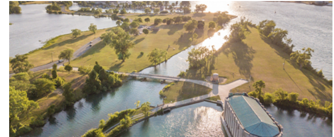
Belle Isle Intake System
