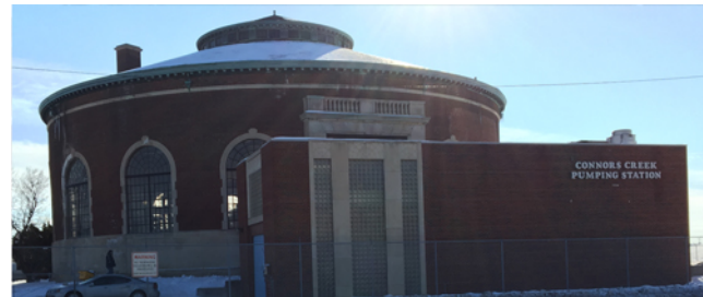
Conner Creek Pump Station Improvements
