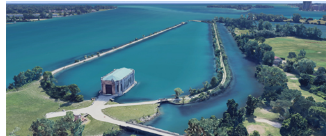
Belle Isle Seawall
