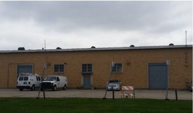
Figure 30: Northwest Pump Station
