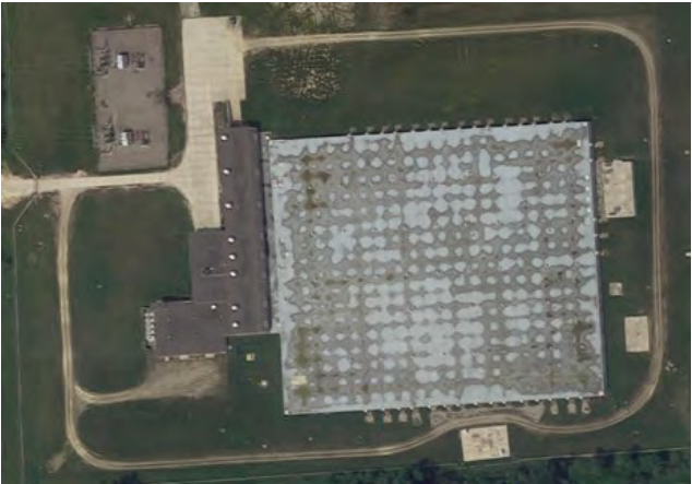
Figure 28. Imlay Pump Station
