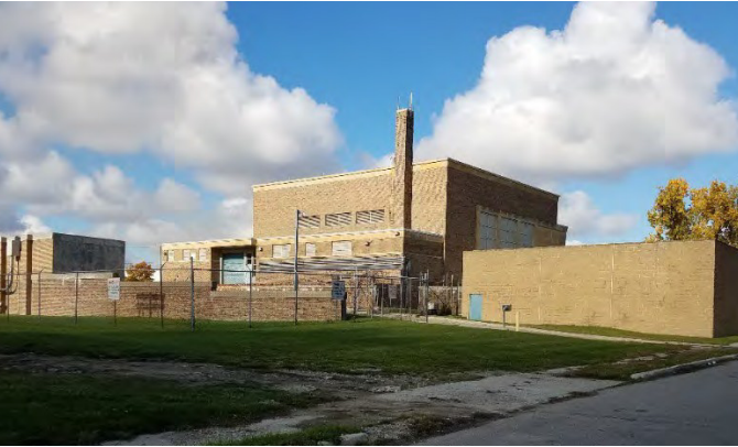
Figure 59. Freud Pump Station
