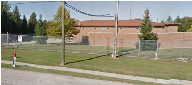
Figure 33. Rochester Pump Station
