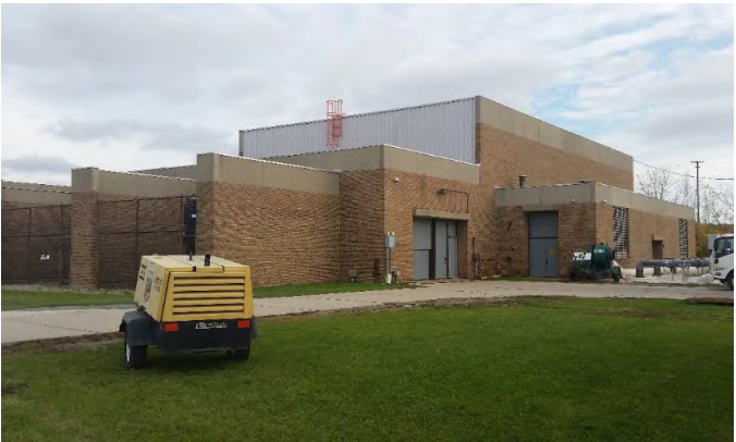
Figure 61. Northeast Pump Station
