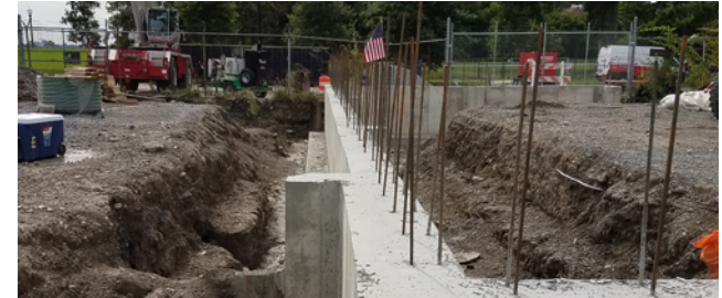
Fairview Pumping Station - Replace Four Sanitary Pumps
