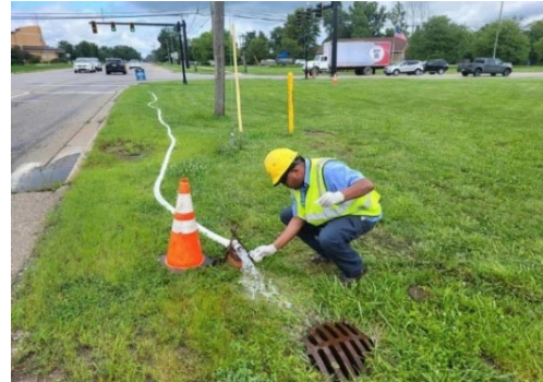
36-inch transmission main
