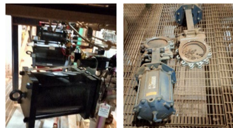
Two of the old Christmas Tree valves removed and three of the new valves installed.
