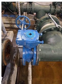
The old De-chlorination Booster Pump #4 isolation valve was removed and the new one installed is shown in the first 2 photos above.
