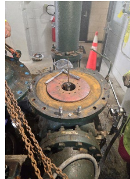
The old De-chlorination Booster Pump #4 isolation valve was removed and the new one installed is shown in the first 2 photos above.
