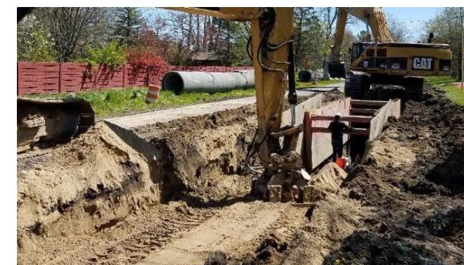
Wick Road 48" Water Transmission Main Construction
