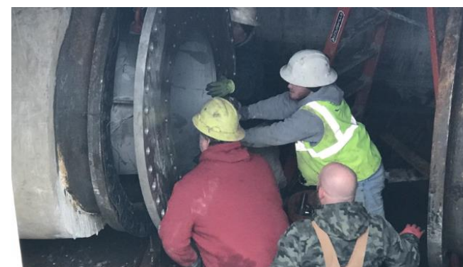
Metering Improvements at Southwest Water Plant
