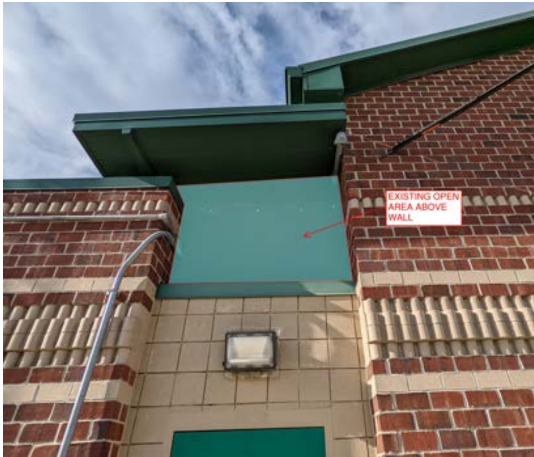
Figure 4-8 Leib CSO SDF – Showing Open Area above West Vestibule partial wall, currently with a bug screen. Similar to the condition at the East Vestibule.
