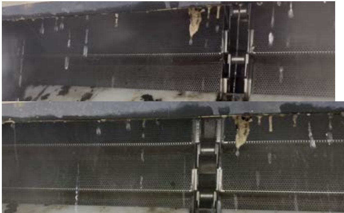
Figure 5-3 – Example of Screen Cleaning with 110 psi Washwater Pressure
