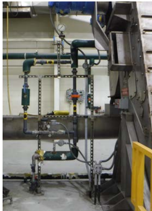
Figure 2-4 Typical Screen Washwater Piping
