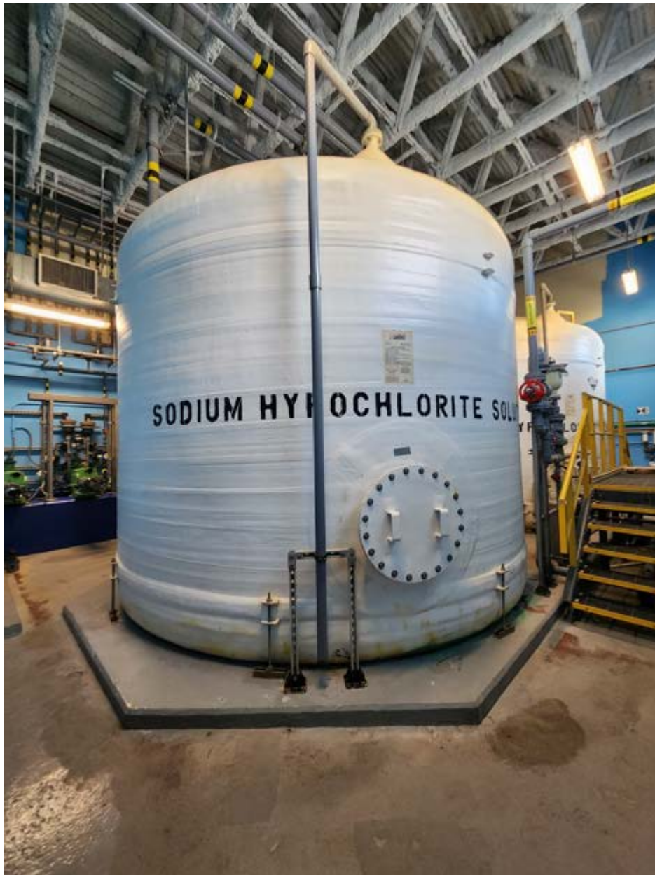
Figure 4-9 Existing Sodium Hypochlorite Storage Tank at Leib
