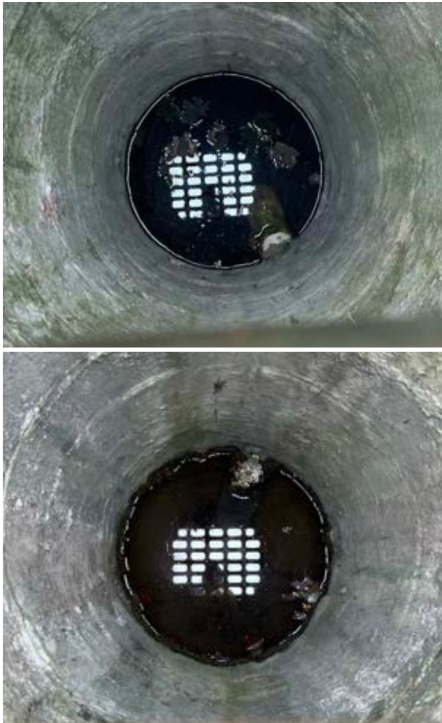
Figure 2-5 Drainage Structures in Alley Adjacent to Leib Facility. Catch basin north (top) and south (bottom) of TTS
