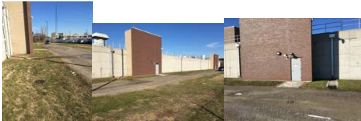
Figure 2-5 Site Photos – East Side of Oakwood CSO Basin
