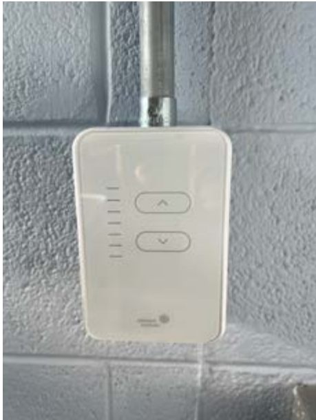
Figure 3-2 Adjustable Wall Mounted Thermostat.
