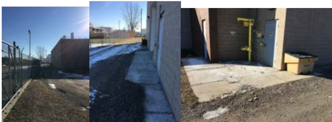
Figure 2-4 Site Photos – North Side of Oakwood CSO Basin
