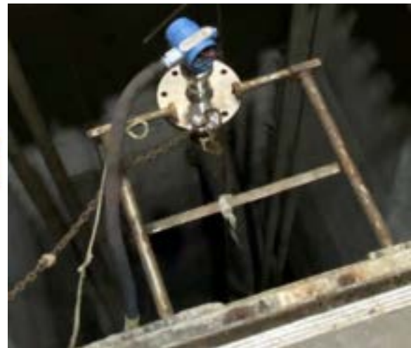
Figure 2-10 Level Sensor Swing-arm Mounting Assembly
