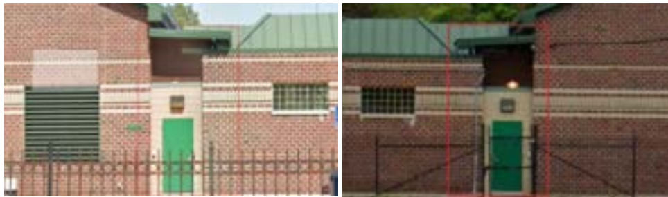
Figure 10-2. Existing West (left) and East (right) Entrance Courtyard
