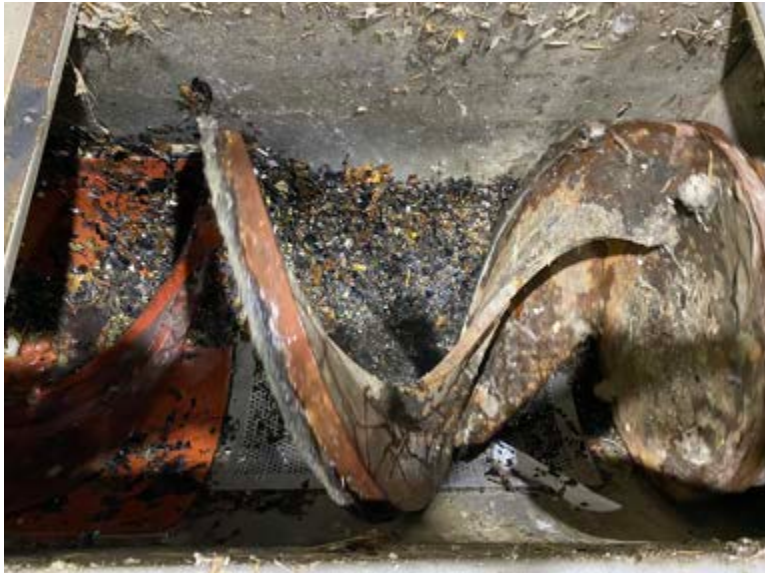
Figure 3-3 Inside conveyor at drain section during operation
