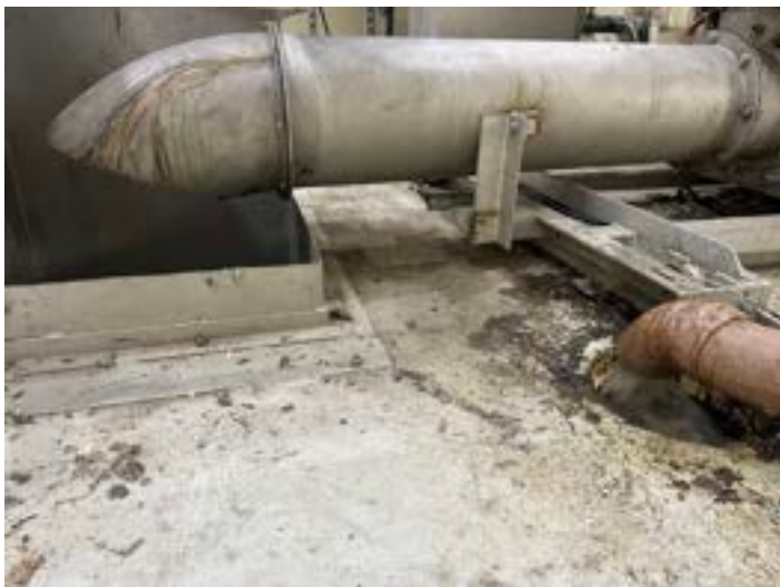
Figure 3-5 Grinder Discharge Tube with Outlet Facing Down (present configuration)
