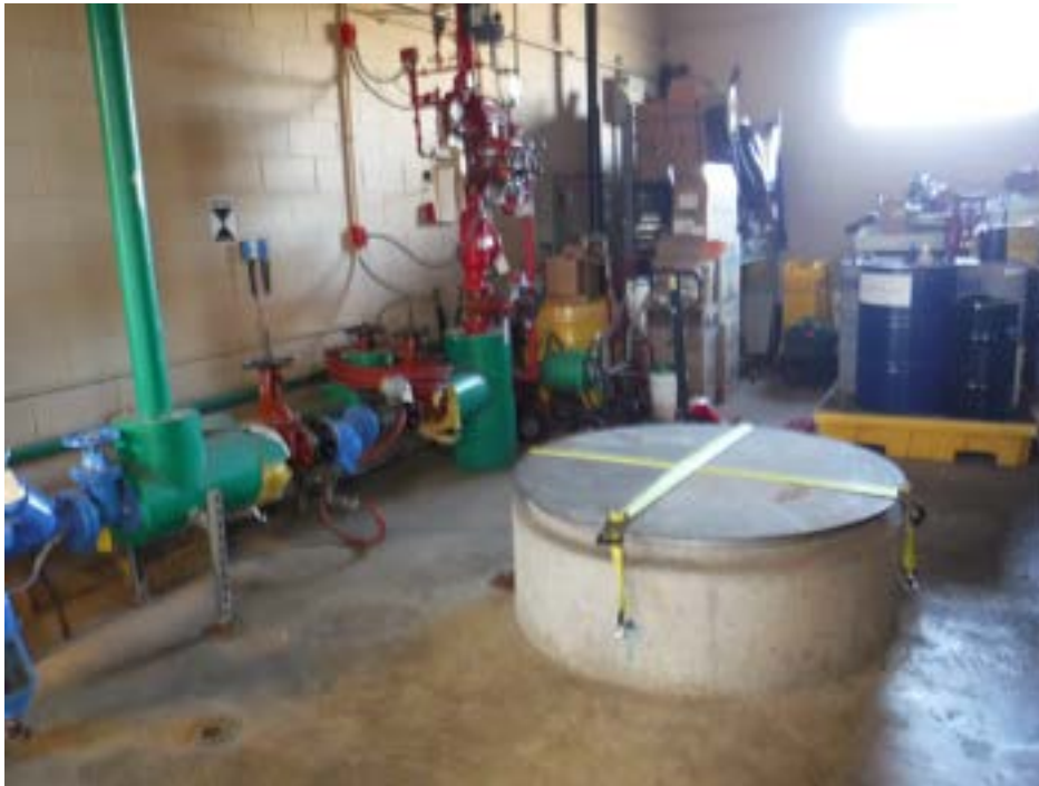
Figure 3-4 Leib CSO SDF – Existing Odor Control Duct penetrating the Odor Control Room (Garage) floor (not used)
