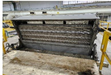
Screen #8 is being rehabilitated
