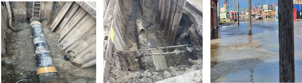
24-inch watermain break at Harper and Hayes
