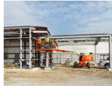
HAZMAT – Steel Structure
