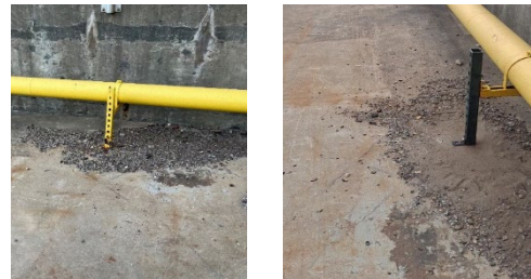
One of the old, corroded pipe supports, and the replaced support prior to painting. The new supports will be painted yellow to match the natural gas piping as shown in the photos
