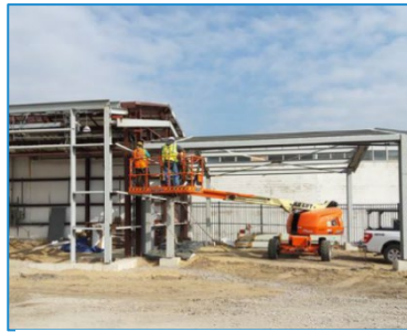
HAZMAT – Steel Structure
