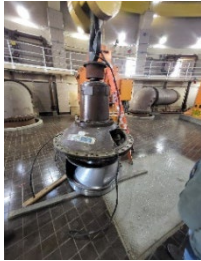
RSP 13 pull-out assembly ready for loading
