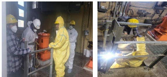
Pictured is Lawrence Lewis, Dakarie Tolbert, Marcus Jackson, and Christina Muscat checking coupling fittings as well as greasing and removing debris.
