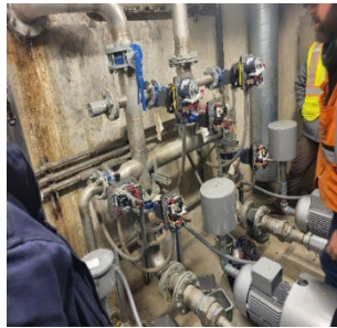
Left is the crew recalibrating valves at in-system storage device (ISD) #5 Lovett Street
