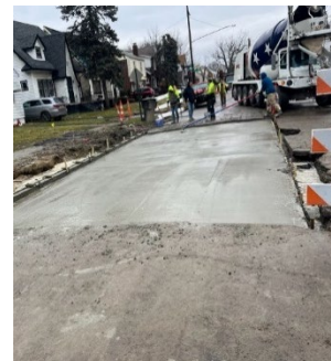
72-inch watermain leak in Detroit: Road restoration
