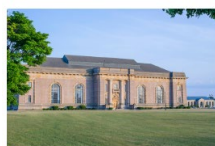
Water Works Park WATER TREATMENT FACILITY
