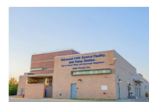
Oakwood Facility CSO & RTB
