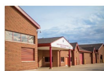
Baby Creek Facility SCREENING, DISINFECTION & CSO
