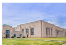
Springwells WATER TREATMENT FACILITY
