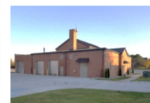
7 Mile Facility CSO & RTB
