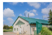
St. Aubin Facility SCREENING, DISINFECTION & CSO
