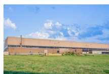
Southwest WATER TREATMENT FACILITY
