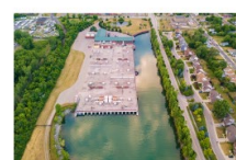
Conner Creek Facility CSO & RTB
