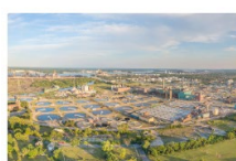
Water Resource Recovery Facility PRIMARY & SECONDARY TREATMENT
