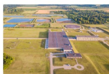
Lake Huron WATER TREATMENT FACILITY
