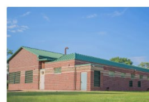
Leib Facility SCREENING, DISINFECTION & CSO
