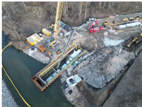
Installation of WTM within Stage 1 of the cofferdam system
