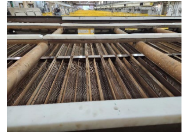
Screen # 15 is being rehabilitated
