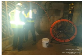
Existing Conduit Investigation
