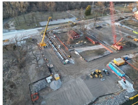
WTM installation entering Avon Rd near the Avon/Dequindre roundabout
