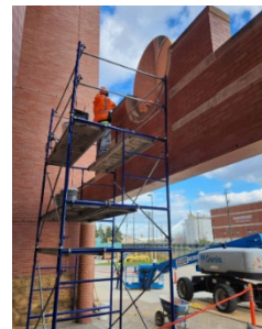
Caulking replacement at NAB
