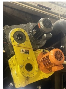
New upper belt installed on BFP
