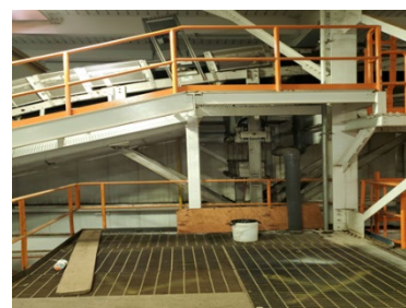
Location of the new access platform
