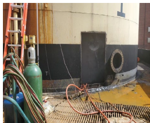
Power Washing to Remove Rubber
