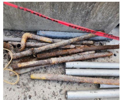
Failed gas line
