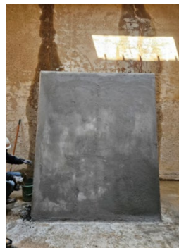
New baffle wall for inlet improvements
