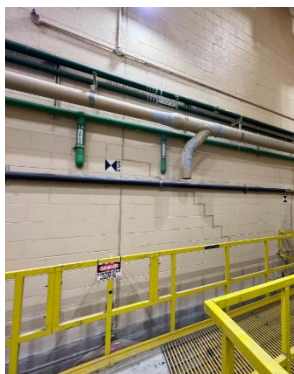
Wall repairs at Puritan Fenkell Facility
