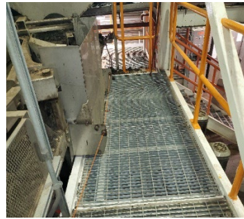
Extended Maintenance Platform at P9 and P10
