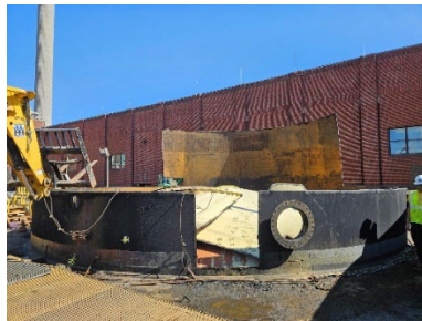
Chemical Building Tank 1 Demolition
