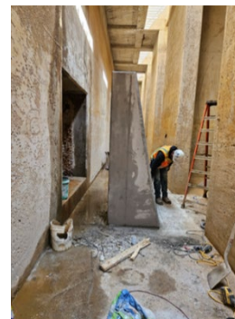
New baffle wall for inlet improvements
