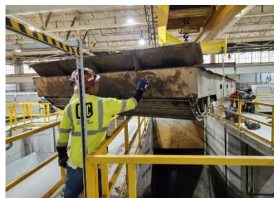
Screen # 4 is being rehabilitated
