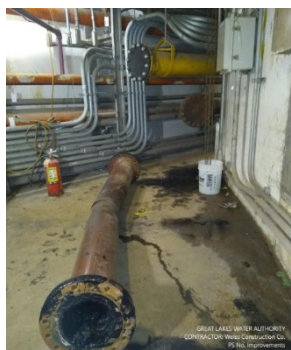
Capped and removal of 10" Sludge line at north end of service tunnel
