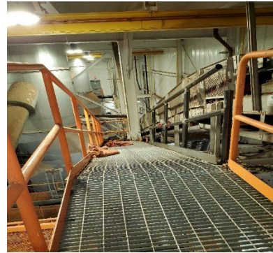
New handrails at conveyor H
