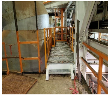
Maintenance Platform at conveyor K and L
