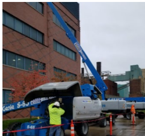
Window caulking replacement at the NAB
