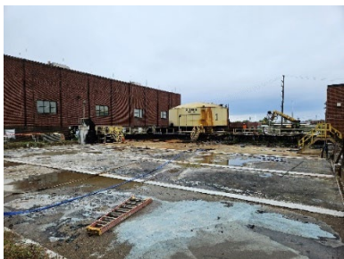
Pickle Liquor Foundation Demolished
