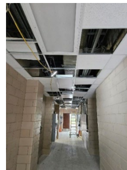
Ceiling and Lighting
