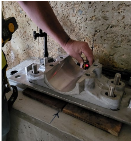
Aligning New Bearings w/ Laser Tracker
