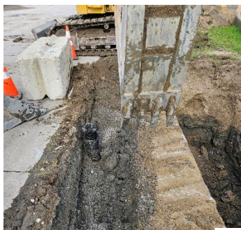
TWAS Mechanical Cleaning Excavation
