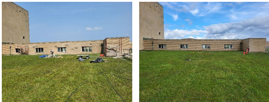
Brick removal and replacement
