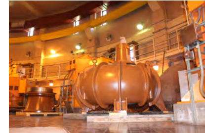
Main Raw Sewage Pumps at Pump Station 2
