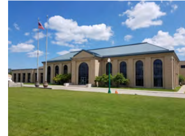
Water Works Park Water Treatment Plant
