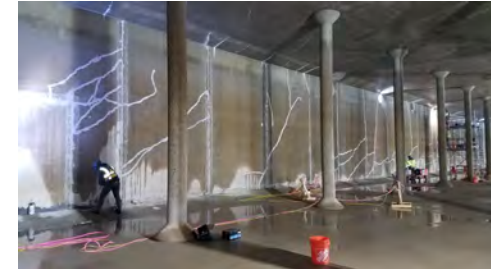
Imlay Booster Station: Sealing interior wall cracks
