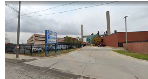
WRRF Front Entrance
