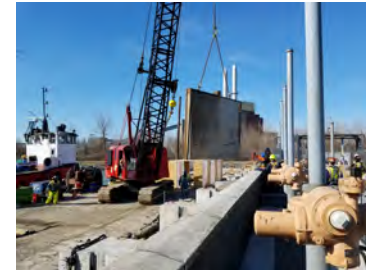
Effluent Relief Gate Repair
