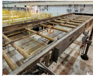
Screen # 3 is being rehabilitated
