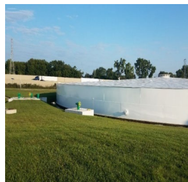
Reservoir #1 Southwest WTP freshly painted
