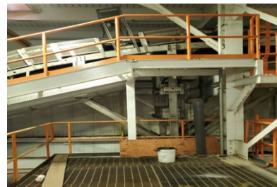
Location of the new access platform
