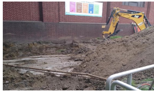
Excavation for a New Electrical
