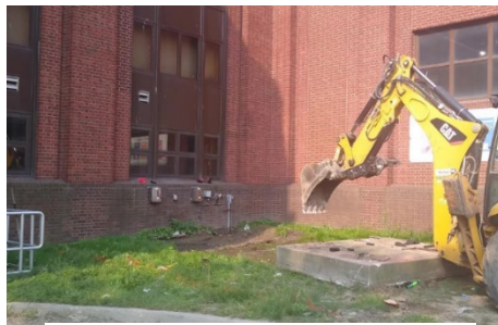
Existing Cooling Unit Pad Removal
