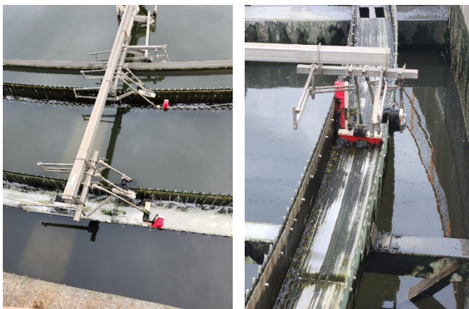
Rehabilitated brush riggings installed on a secondary clarifier
