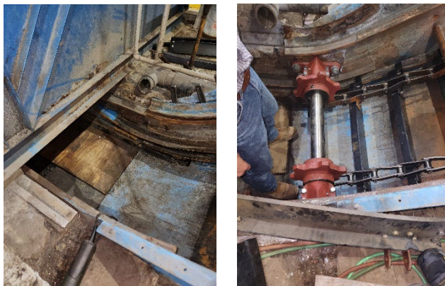
The inflection point of Grit Flight 1 where the flights start moving up to move grit to another conveyor. These pictures are before and after the sprocket installation.
