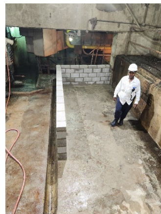
Operations Team Leader Joseph Rowland, looking at the newly constructed containment wall in the Pump Station 1 basement
