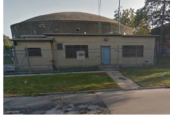
Figure 22. Electric Avenue Pump Station
