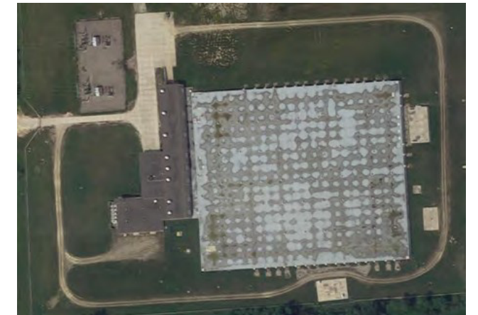
Figure 28. Imlay Pump Station
