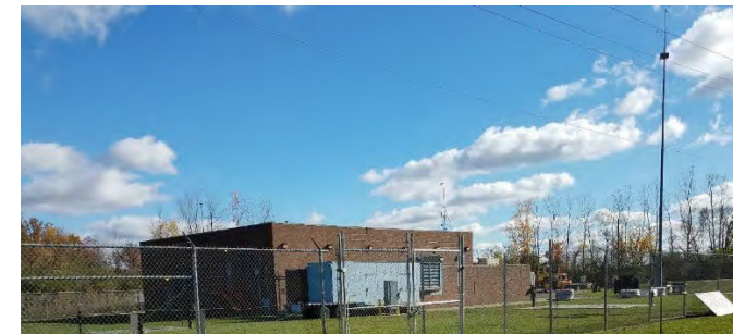
Figure 38. Ypsilanti Pump Station
