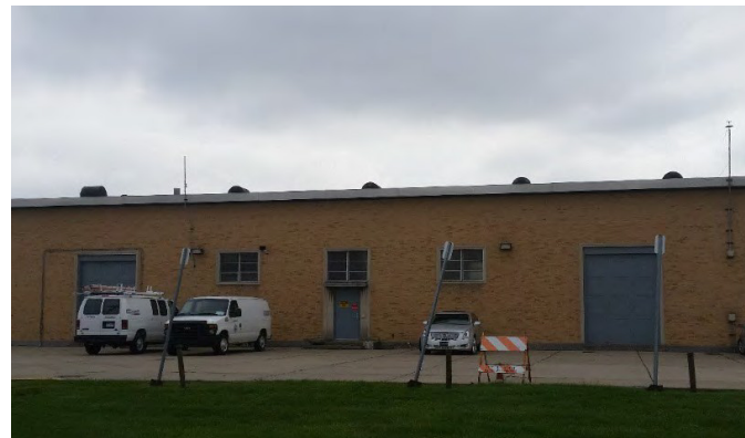
Figure 30: Northwest Pump Station
