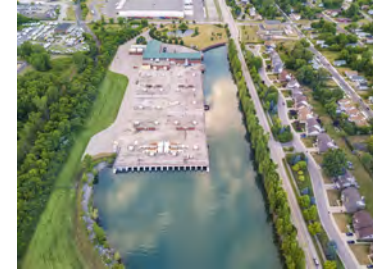
Conner Creek CSO Facility
