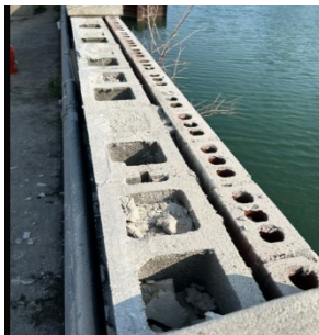
Capstones repairs at CON
