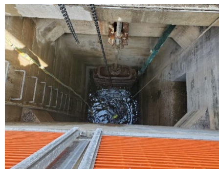
Flap gate being installed
