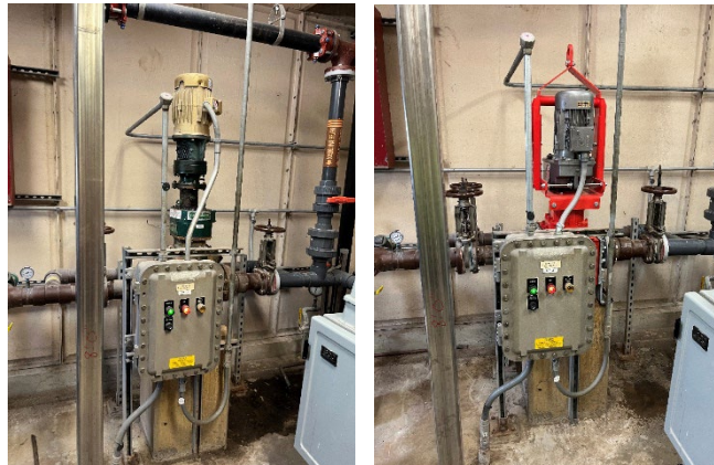
The old grinder faced similar clogging issues experienced with the belt filter presses and has been replaced with a more modern model
