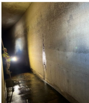
PC#18 Effluent Channel Assessment
