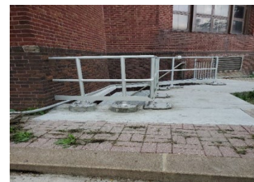
Task 2J-01 Upper Wet Well Stairwell
