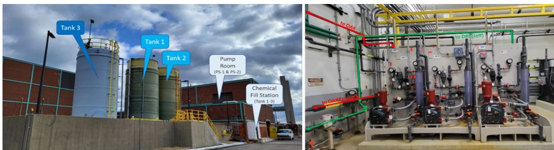
Ferric Chloride system at Pump Station 2 servicing both pump stations (left) Pump skid feeding to Pump Station 1 in the Pump Room (right)
