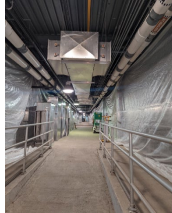
Newly installed ductwork in rapid mix area
