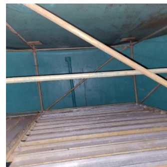
Inside of Baby Creek chemical tank #2; new spray on liner with scaffold for further spark testing.
