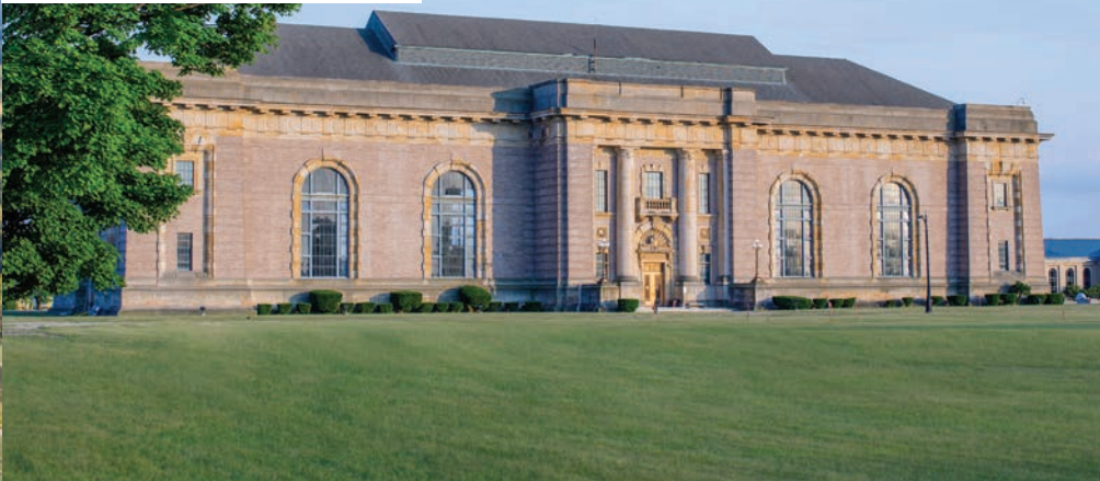
WATER WORKS PARK
