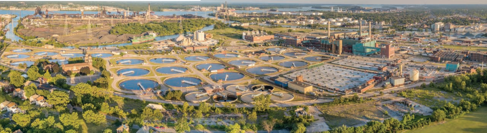
WATER RESOURCE RECOVERY FACILITY
