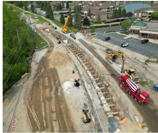
96-inch WTM installation on Dequindre Rd. north of 23-mile intersection
