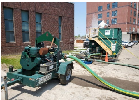
Chemical Cleaning of permanent TWAS line
