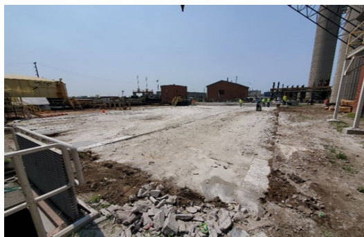
Three Ferric Chloride Tanks Removed
