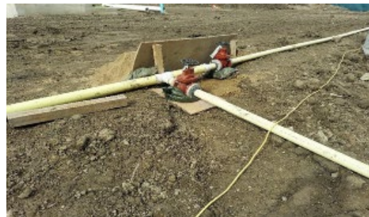
4-inch temporary main for pressure testing
