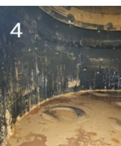
Tank #2 lining - Bubbled gasket lining
