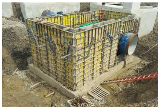
Formwork for valve vault V-06
