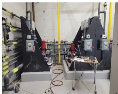
PS-2 Ferric Chloride Pump Skids
