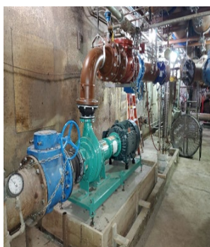
Task 70 Complex A Gallery SFP-2 Pump Replacement
