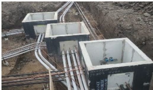
Duct bank installation near venturi meter M-06
