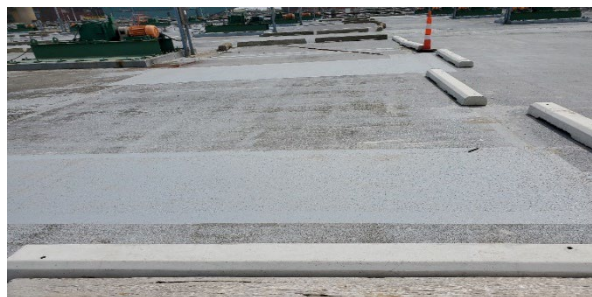
Newly installed planks under task J2-05
