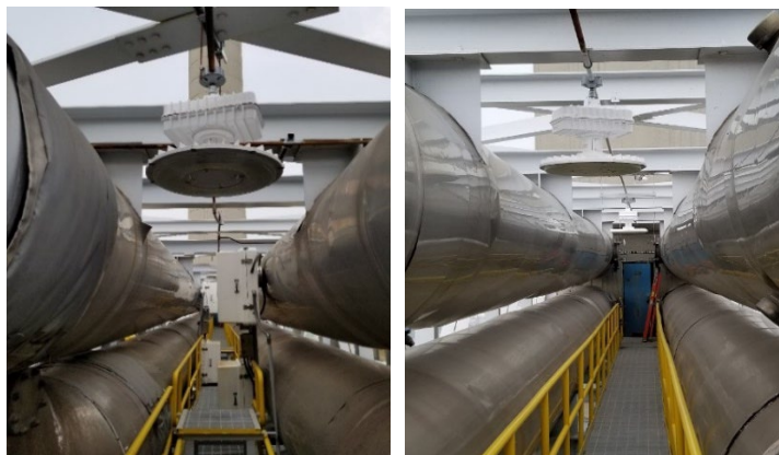
New light fixtures installed on the catwalks to the tall stacks at WRRF
