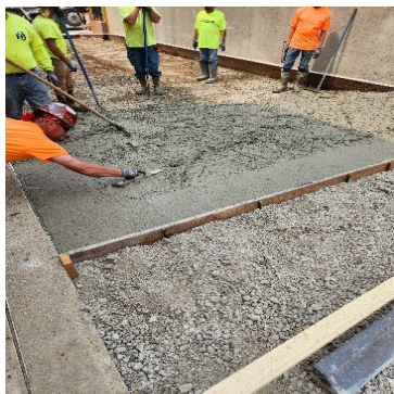
New Concrete West of Chemical Building
