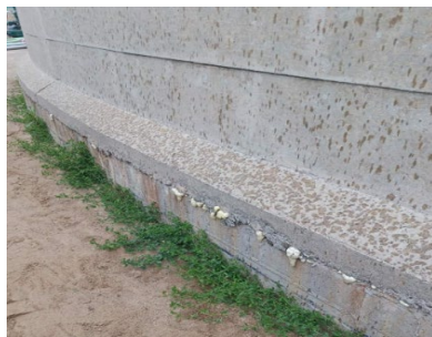
STT-14 Leak Repairs
