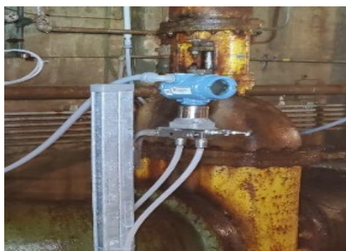
NEWTP new loss of head meter (Typical 1 of 88)
