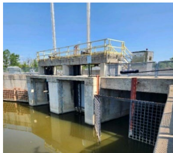
Shunt bypass emergency gates at Hubbell-Southfield
