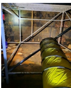
Scaffolding inside of Tank #2 at Baby Creek
