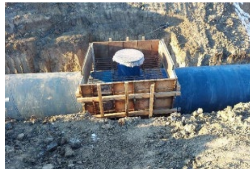
Air release valve foundation formwork
