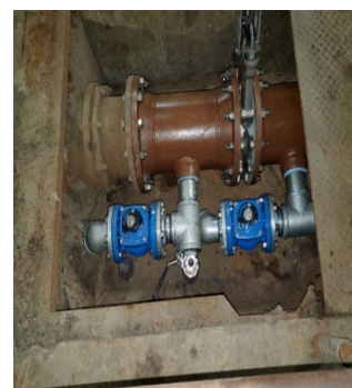
Task 70 SST No. 1 and 3 Equalization Valve
