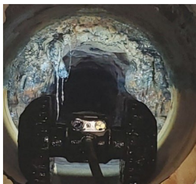
Vivianite Remaining in TWAS Line after Initial Chemical Cleaning
