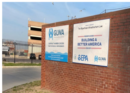
Project signs installed are shown above
