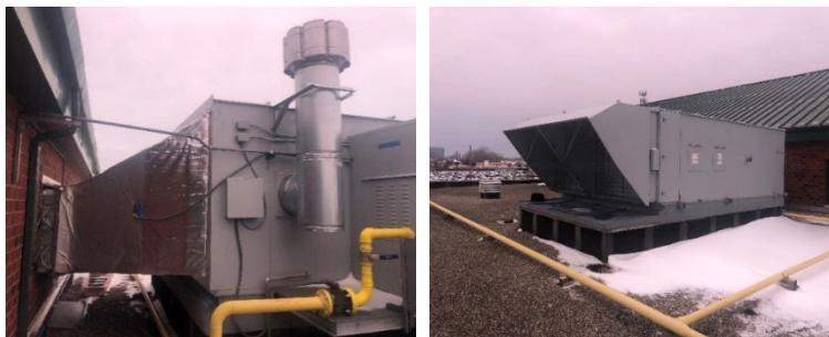
The newly installed makeup air unit-2 is shown in the left and right
