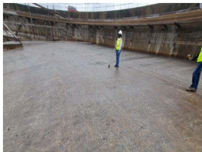
Primary Clarifier 17 Assessment
