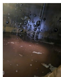
The discolor of NaOCl shows chemical is behind the liner
