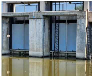
Shunt bypass emergency gates at Hubbell-Southfield
