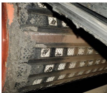
Failed Conveyor Drive Pulley
