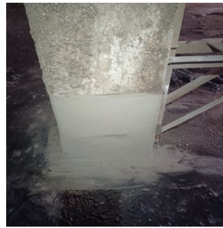
Spall repairs at HS Basin
