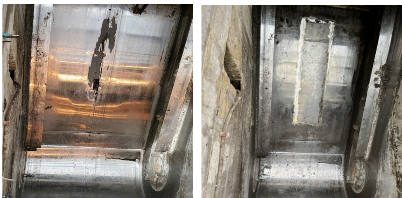
Photos above show the scum collector trough before and after the new plate was welded
