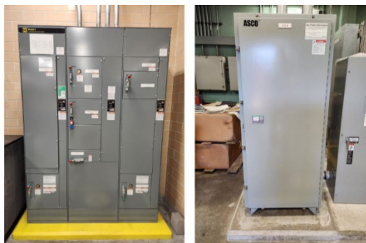
Figure 2: The new motor control center (EMCC-2B-10) and automatic transfer switch (ATS-2)
