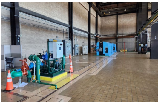
Figure 2: The booster pumps (foreground) and raw water screens (background) including level monitors and control panel
