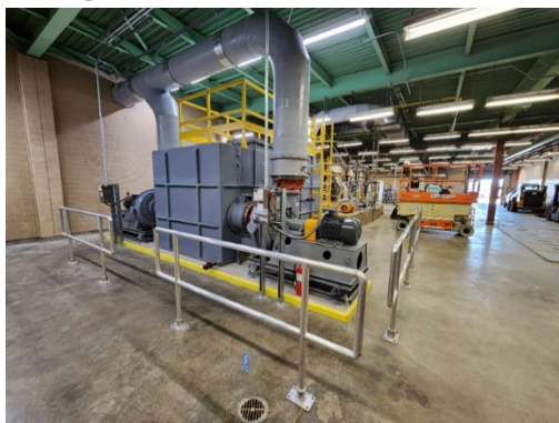
Figure 3: New chlorine scrubber system including ductwork and blowers
