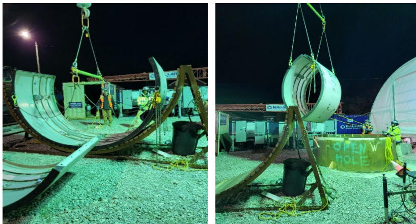
Two of the three sections that make up one ring being lowered into access shaft
