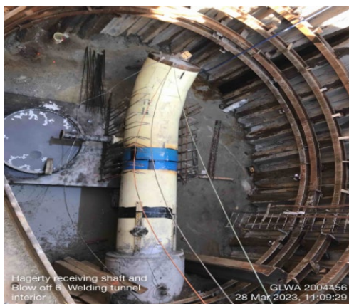
A look down inside of the receiving shaft
