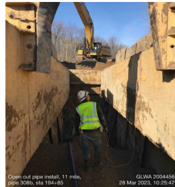
Trenches for open cut pipe installation
