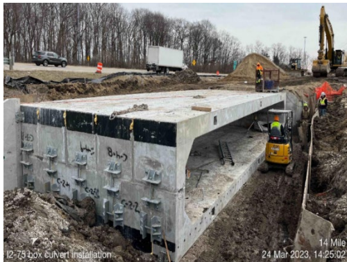
Installation of box culvert on I-275 bike path
