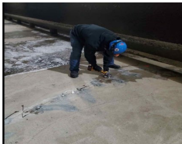
Crack repairs at 7 Mile
