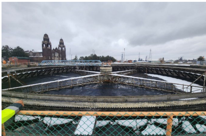
Secondary clarifier B-19 drained and cleaned for rehabilitation pictured above
