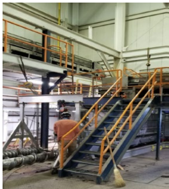
Screw Hopper 14A Auger Repairs
