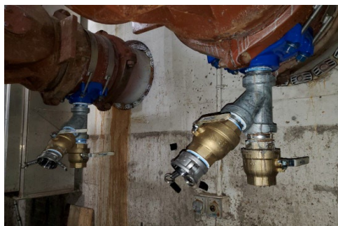
New 3-inch diameter drain lines installed for the 18-inch diameter Sludge Feed Piping for Sludge Storage Tanks 5 and 6, JOC Task 70.JOC Task J2-01
