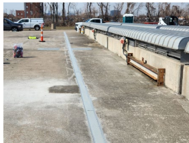
Expansion Joint Repairs at CON
