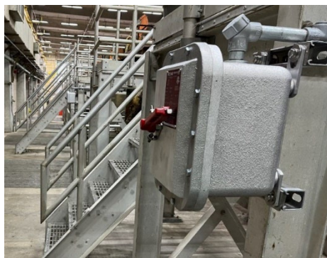
New local disconnects installed for the bar racks at Pump Station 2
