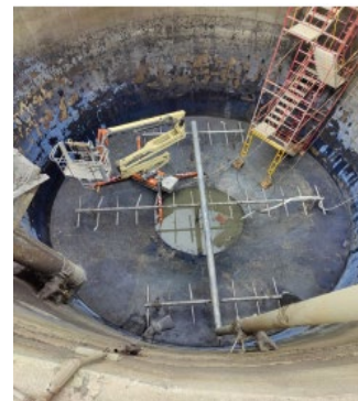
NAB water leak repair
