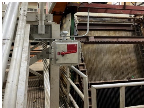
New local disconnects installed for the bar racks at Pump Station 2
