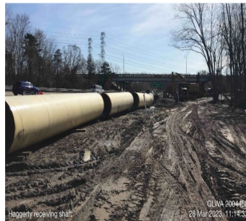
Pipe stage for installation along Haggerty Road
