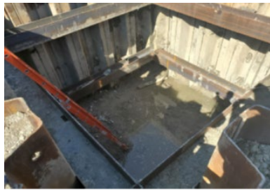
Jack/Bore Receiving Pit Excavation
