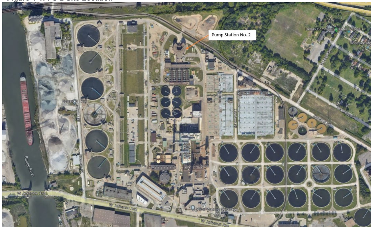
Figure 4-1: PS-2 Site Location
