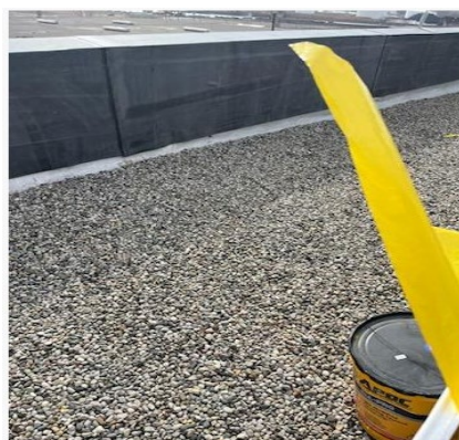
NAB water leak repair
