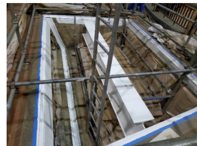
View of opening after painting
