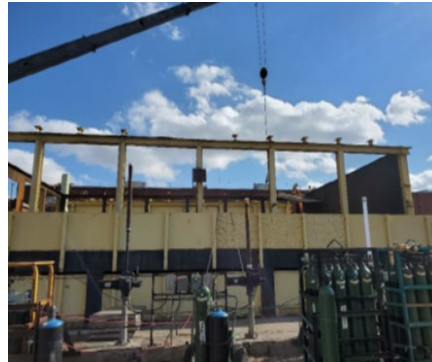
Ferric Tanks Demolition
