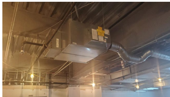
Fan Powered Variable Air Volume (VAV) installation in progress
