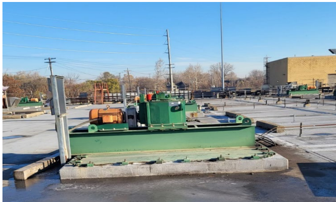
The image above shows mixer 3-7-B with a new gearbox installed. The vibration monitoring report showed the gearbox for the mixer was near failure.
