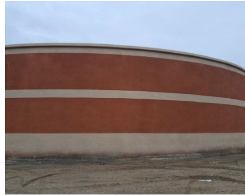
Completed Exterior Coating on Reservoirs
