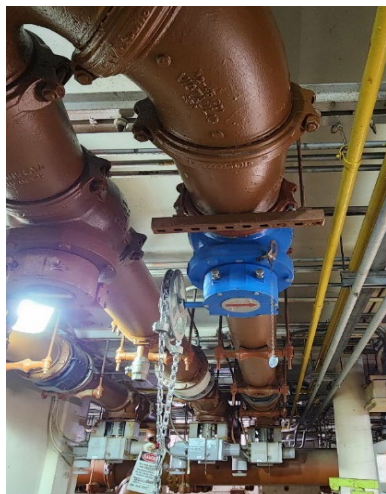
One of the replaced valves and the secondary water line connection at the east wall shown in images above.
