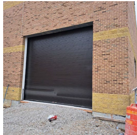
Overhead door installation complete on new pump station
