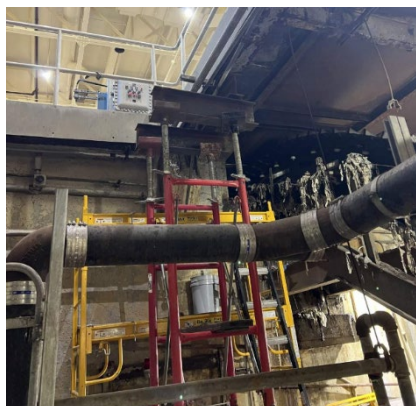
PS-1 Rack & Grit – Corbel Repairs
