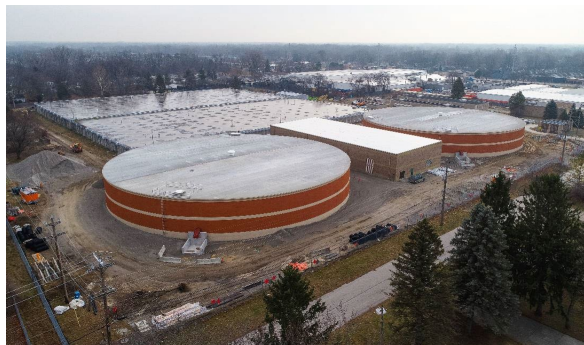
West Service Center Pump House and Divisional Valve Replacement Project view from northwest corner
