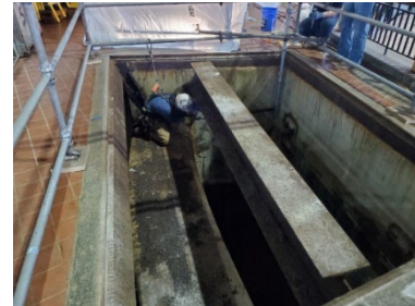
View of opening as scaffolding is installed prior to painting
