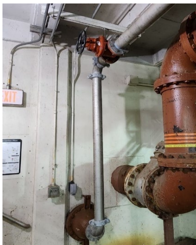
One of the replaced valves and the secondary water line connection at the east wall shown in images above.
