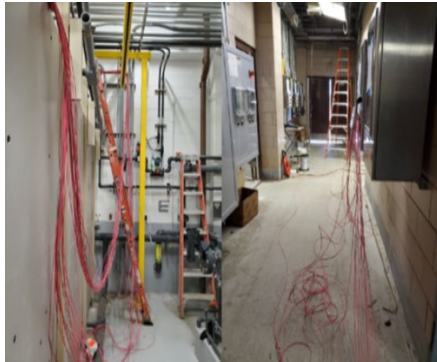
Wiring Installation in the Chemical Building
